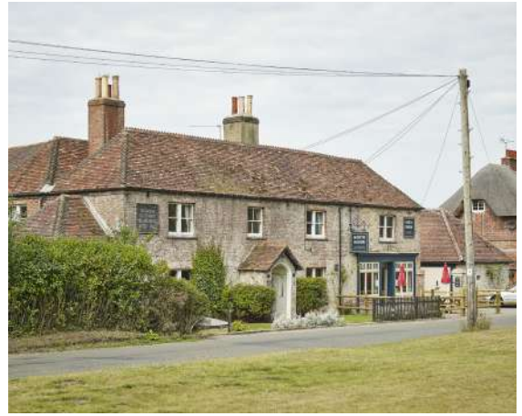
Northbrook Arms, East Stratton
