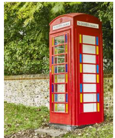
K6 Kiosk at St James church Woodmancott
