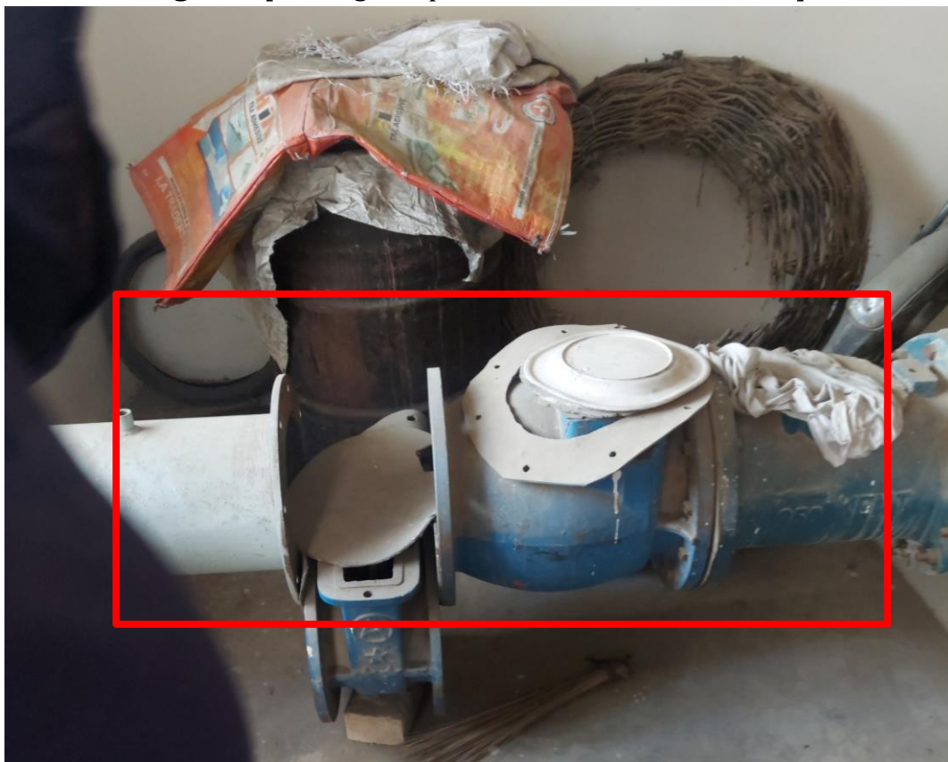
Figure 5 [Missing valves]
