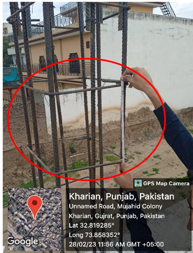
Figure 5: Wider Stirrup Spacing at Lap Splice
