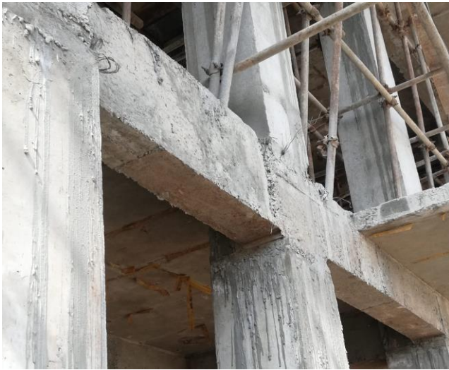
Figure 5: Eccentricity in Beams
