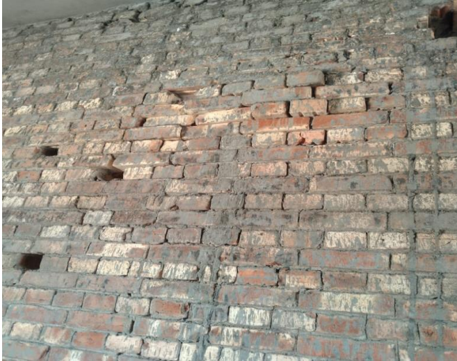
Figure 1: Poor Mansory Work
