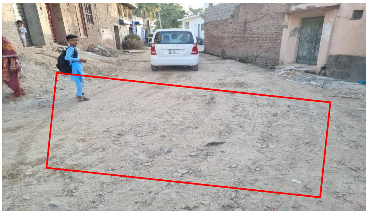
Figure 4: Un Constructed Portion in Between Constructed Road
