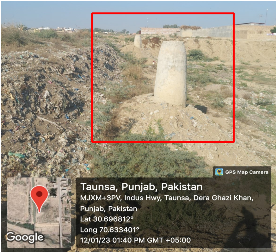
Figure 8 [Manholes without any Later Support/Backfill ]
