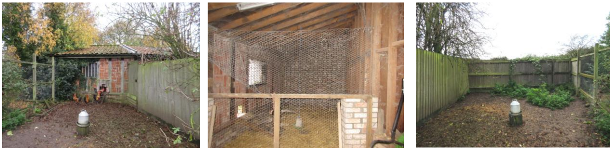
Compartment 1: Left: external elevation looking SE; Centre: interior looking NE; Right: associated enclosure looking NW
