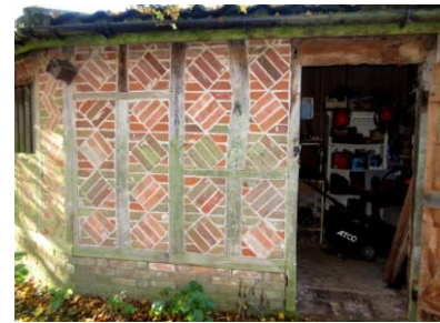
Left: interior looking NW; Centre: NE elevation of compartment 10; Right: doorway and diamond pattern brick nogging of E elevation of compartment 9
