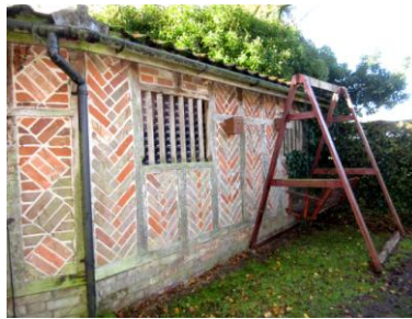
Left: interior looking NW; Centre: NE elevation of compartment 10; Right: doorway and diamond pattern brick nogging of E elevation of compartment 9
