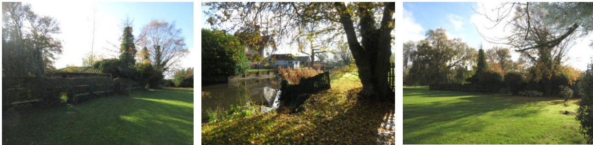
Left: looking SW towards outbuilding from lawned area; Centre: looking SE across the moat from the outbuilding; Right: looking S towards the outbuilding from the lawned area NW of the Hall
