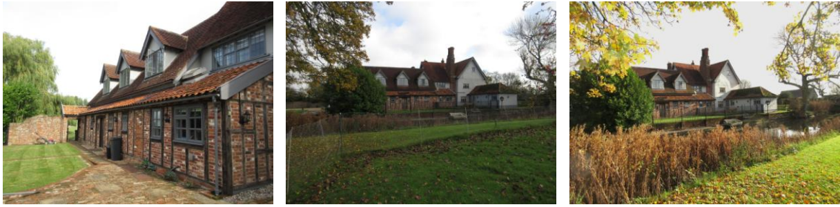
Left: W elevation of W wing showing brick nogging similar to the outbuilding; Centre: looking SE from grassland to S of outbuilding; Right: looking SE from outbuilding towards the Hall
