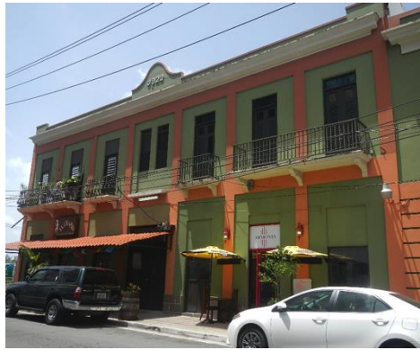
Figure 81. Tenement-house building, Puerta de Tierra Historic District, San Juan de Puerto Rico, 1922, Block 141 Parcela 08 and Parcela 09, 2017. APC.
