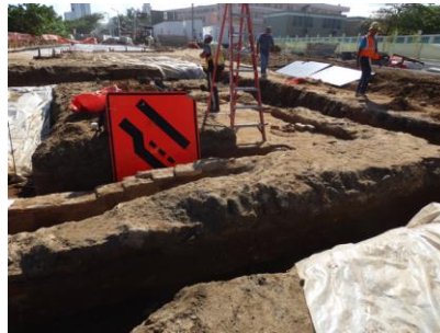
Figure 39. Excavations during the construction of the Paseo de Puerta de Tierra, Puerta de Tierra Historic District, San Juan de Puerto Rico, 2014-2015, Mr José López.
