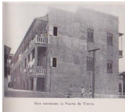
Figure 77. A Puerta de Tierra tenement-house described in 1926 as a “new” construction. Knowlton Mixer, Porto Rico History and Conditions Social, Economic and Political .
