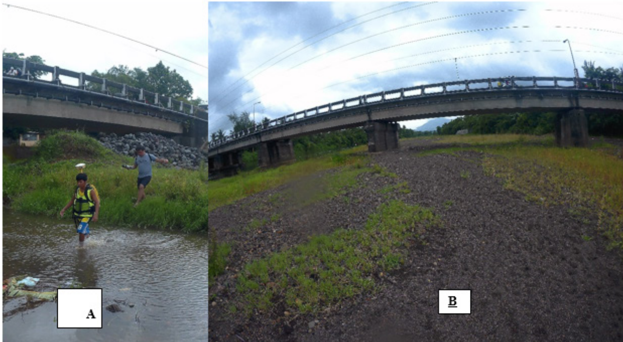
Figure 35. A) Cross-section survey in B) Imperial Bridge facing downstream
