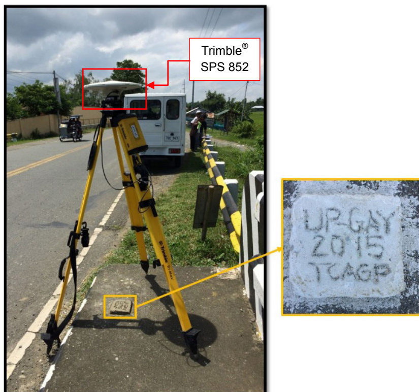
Figure 32. GNSS base receiver setup, Trimble® SPS 852 at UP-GAY in Gayaga Bridge, Alaminos City, Pangasinan
