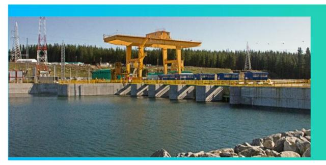
34MW run-of-river, 14Mm3 reservoir ~60km of Los Angeles, Bío-Bío. Operating since 2015. Powerhouse w/2 17.2MW Bulb-Kaplan units 26 mt-high concrete dam, 5 spillway radial gates, 2 gantry cranes Connected to SEN @ El Rosal SS. 17-km T line from Laja SS
