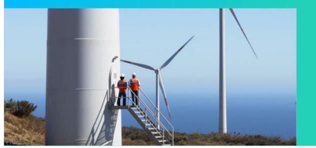
48 MW (24 Vestas V90 WTGs(\*), 80m hub height, 90m rotor diameter, 125m total height) 1,000 hectare site in Coquimbo region In operation since 4Q-2009
