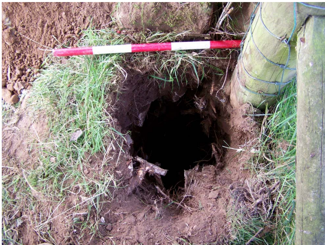
Plate 9: New posthole excavated to the north of Site 3, looking south
