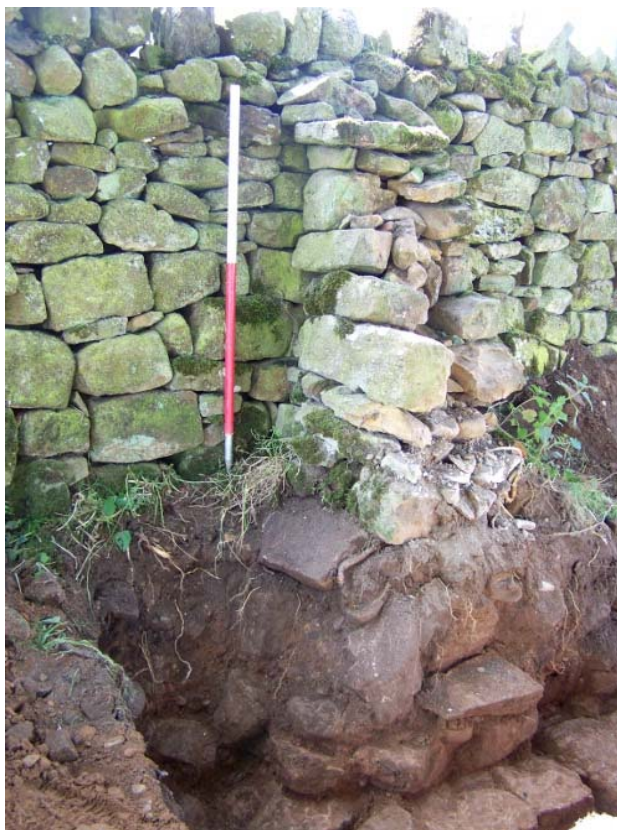
Plate 7: Boundary wall 302, sitting directly upon Hadrian's Wall (303), looking south-west
