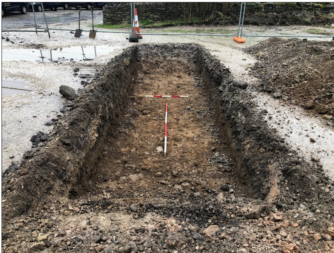
Plate 1: Trench 1, looking east with 2 x 2m scales
