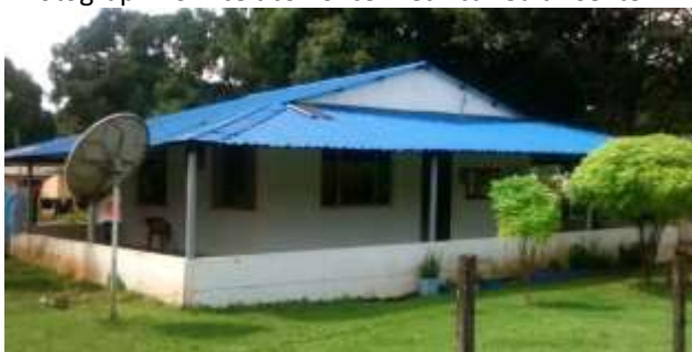
Photograph 43: Aceitico Police Precinct Health Center
