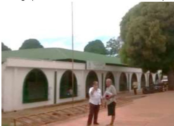
Photograph 22: E.S.E. location San Juan de Dios Department Hospital
