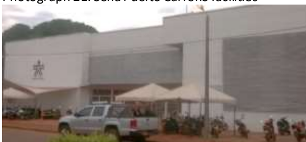
Photograph 21: Sena Puerto Carreño facilities
