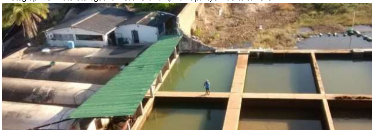
Photograph 19: Water Storage and Treatment Plant, Municipality of Puerto Carreño
