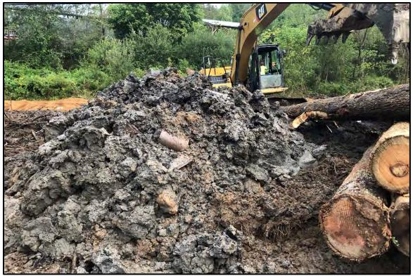
Figure 6.4. Hydric soils and terra cotta pipe fragments in UT-1.
