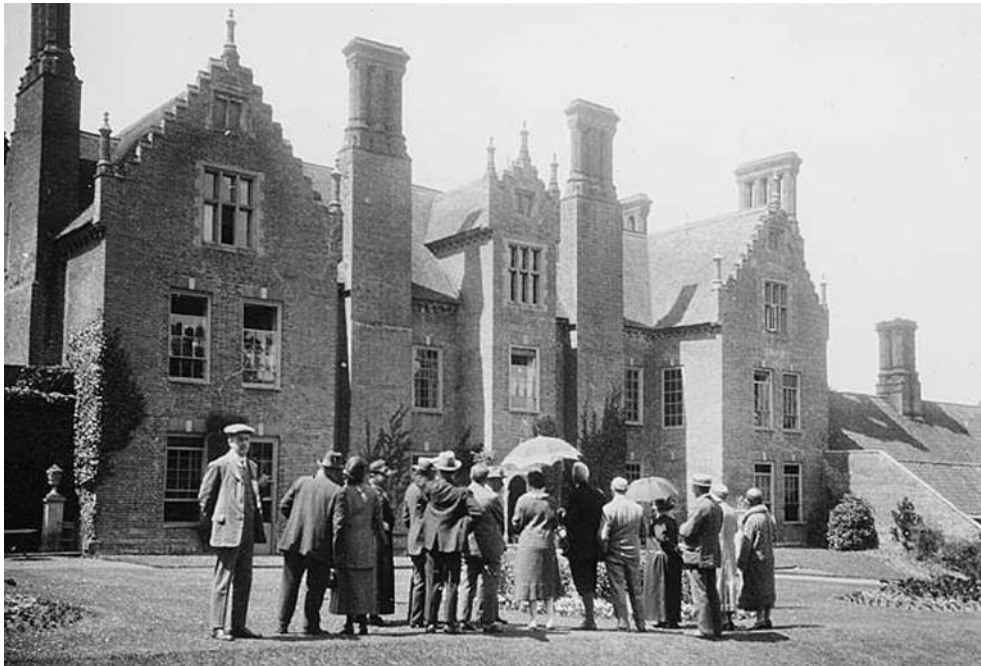
Fig. 4. Spixworth Hall, Norfolk (dem.), built 1609, rear façade, 1925 photograph. English Heritage, National Monuments Record.
