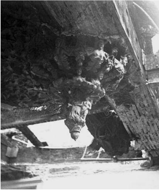
Fig. 6. Merton Hall, Jacobean plaster ceiling pendant, modelled with The Fall of Man , in first-floor 'Adam and Eve Room' or Great Chamber, post-fire photograph, 1956. Allan Sewell .
