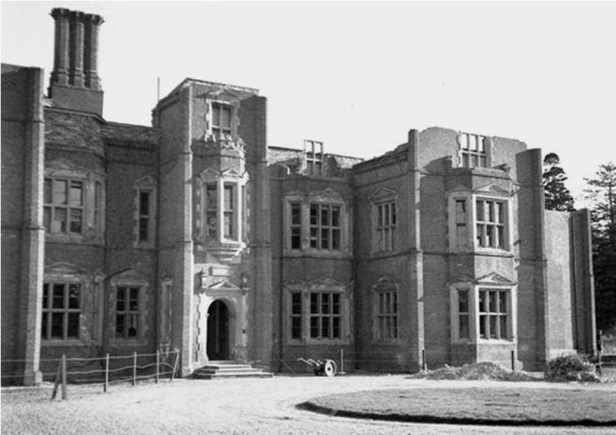
Fig. 23. Merton Hall, entrance front in post-fire stabilised form, from north-east, 1956.
