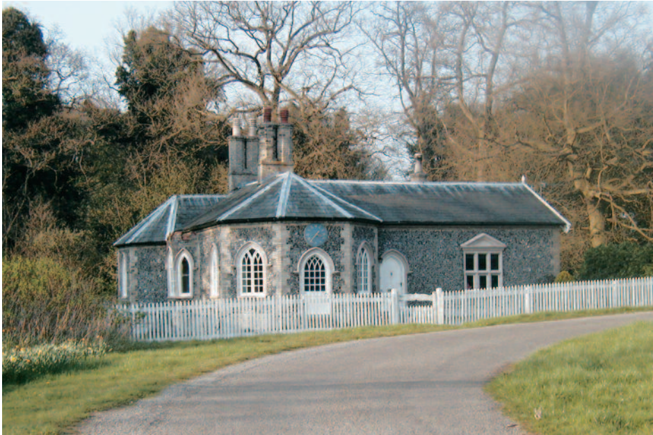
Fig. 17. Merton Hall Lodge, of split flint and gault brick, c.1828, here attributed to Fuller Coker of Shipdham, Norfolk. Richard Garnier .
