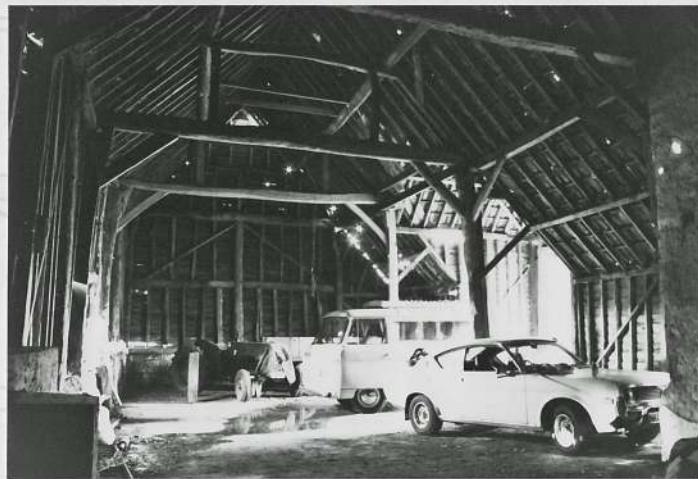
Barn, looking east, corner of cob wall on the right
