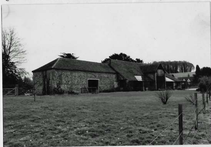
Converted barn & attached b.s.f. building, west side.
