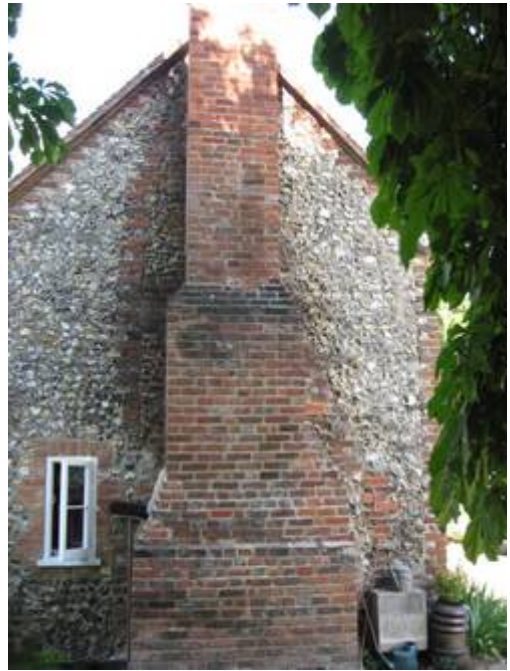
South gable end stack
