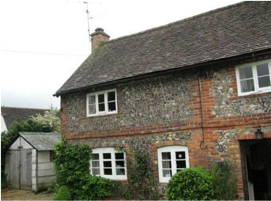
Front east elevation, showing the straight brick join between the earlier, l.h. building and the extension to the right. The flat brick arch over the door is probably a modern repair.
