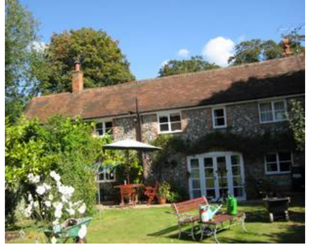
Front, south elevation. The one-bay original cottage is on the left, the area to the right of the down pipe is C20 th .
