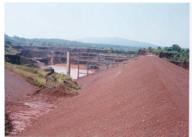
The addition of chemicals for faster settling of suspended solids also binds the sludge and hence, increases life of the slime dam.
