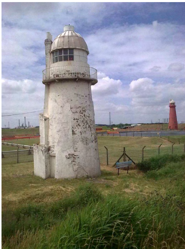
Plate 1: Lighthouses A42 (foreground) and A41; looking west towards application area
