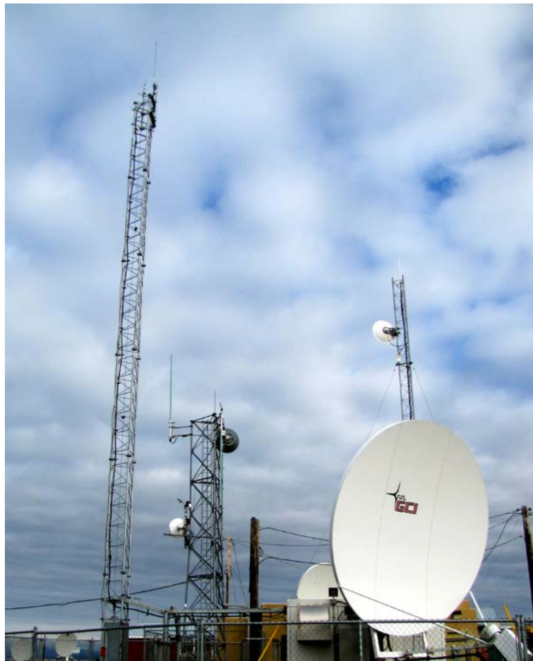
Communication Towers in Teller
