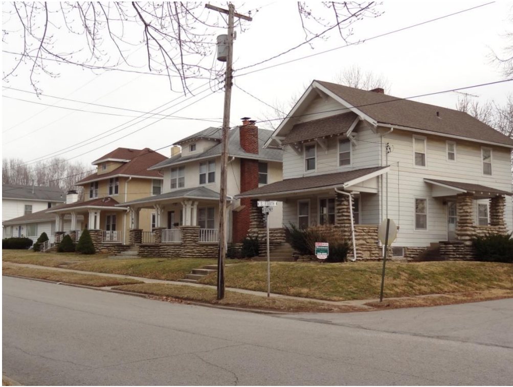
300 Block W. Broadway, looking southeast
