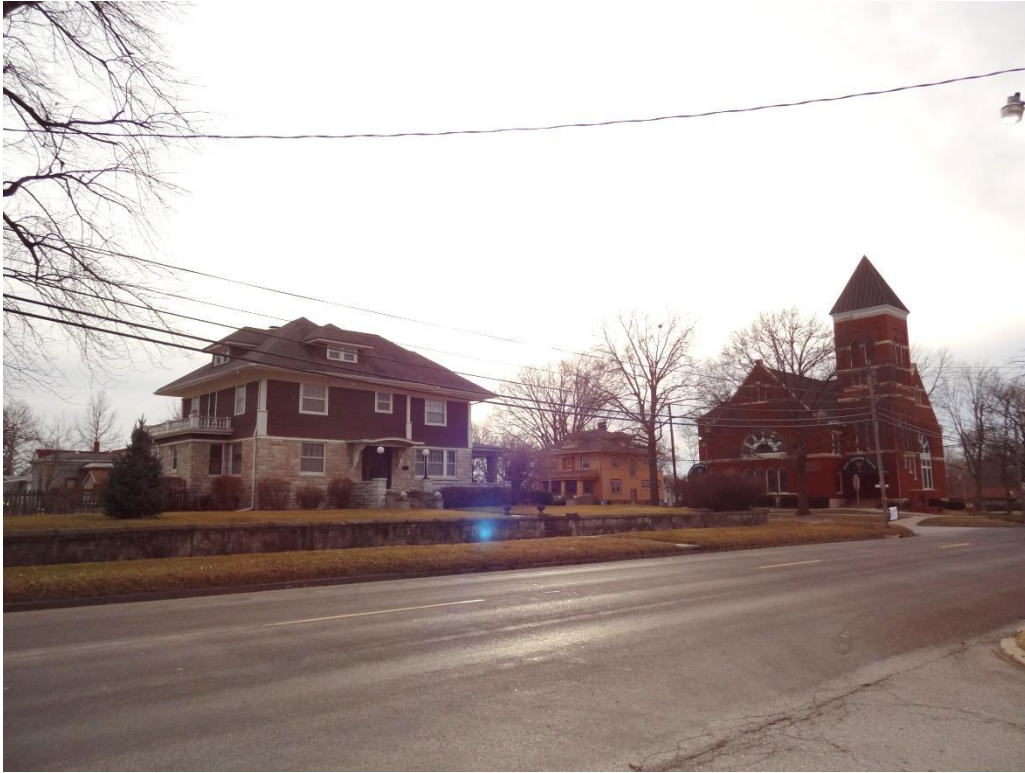
Intersection of W. Clay & Birch, looking southwest.
