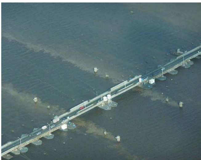
Demerara Harbour Bridge
