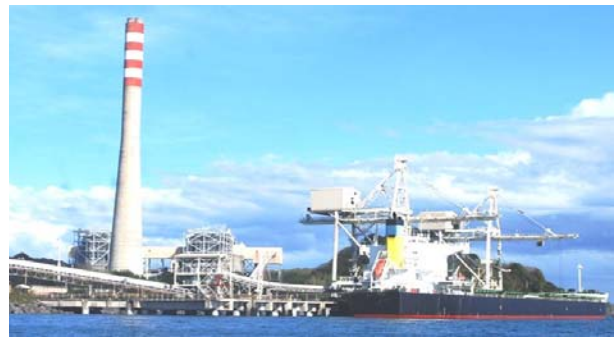
Pagbilao Power Station—Coal Berth
