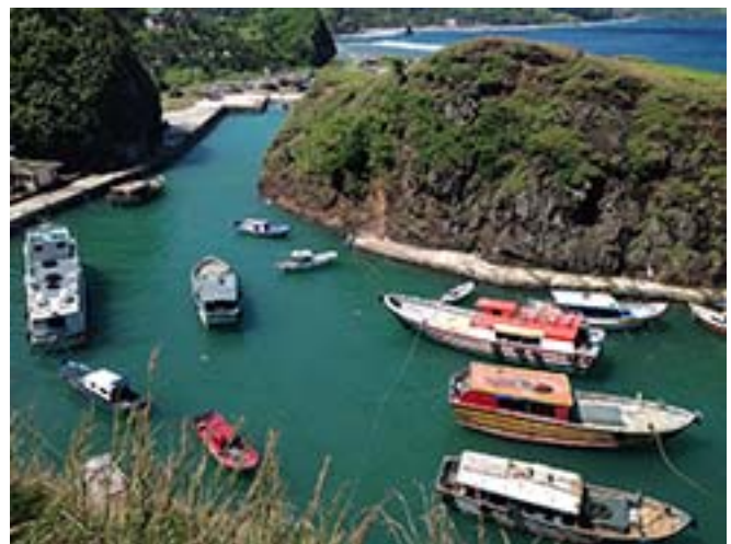
Mahatao Boat Shelter
