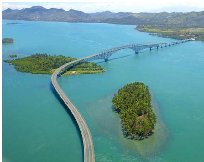
The San Juanico Bridge connecting Samar and Leyte
