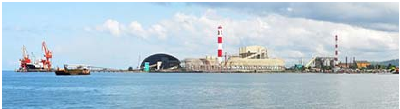
Toledo Harbor—Toledo Power Company Wharf
