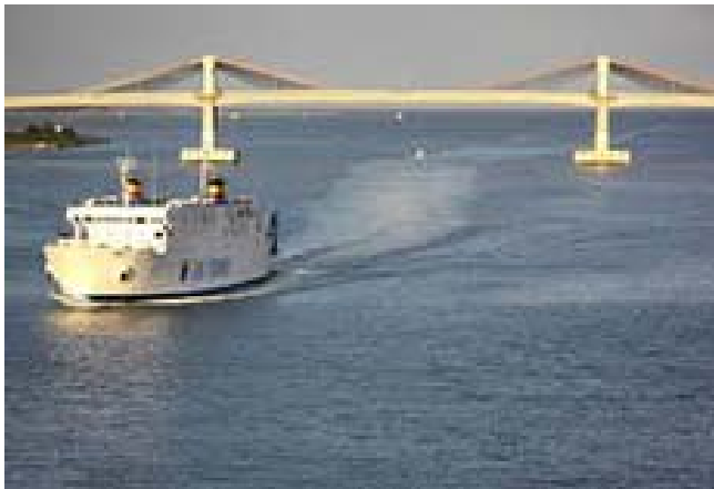
The Marcelo B. Fernan Bridge (Mactan Bridge)
