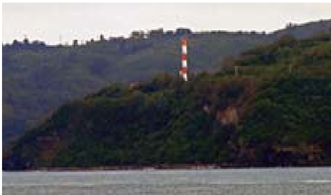
Batangas VTMS Radar Station
