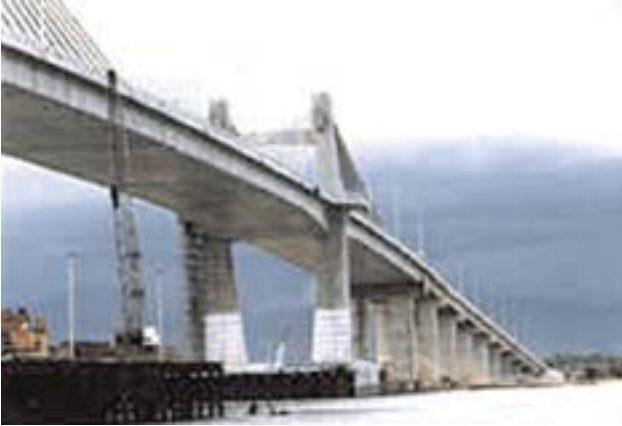
The Marcelo B. Fernan Bridge (Mactan Bridge)
