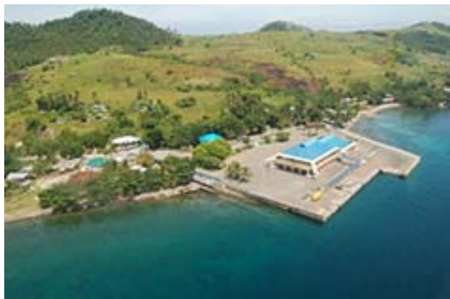
Lipata Ferry Terminal
