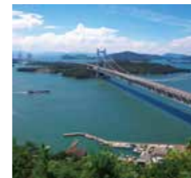
Seto Ohashi Bridge
