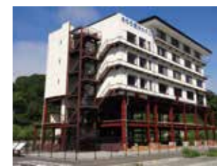
Post-tsunami remains of the Taro Kanko Hotel
