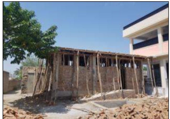
Fig. 24. Shuttering for beams/slab in progress at LB - GPS Hawaii, Nowshera
