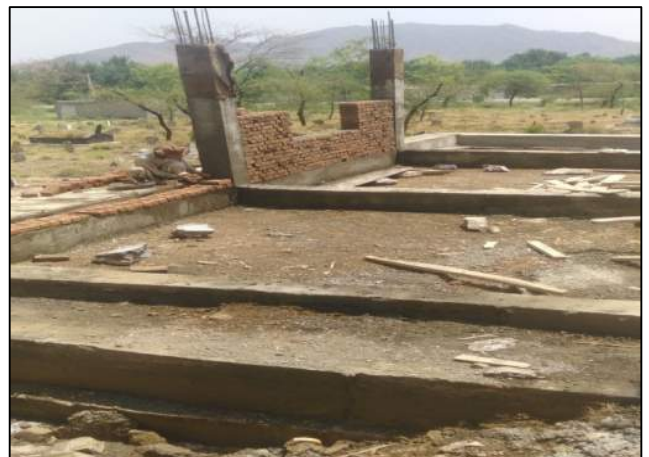
Fig. 60. Brick work was in progress on M-2 Gulzada Kalay, Malakand
