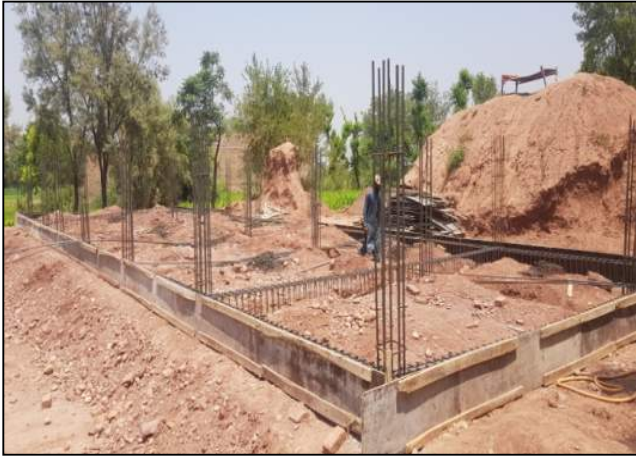
Fig. 31. Formwork fixing in progress-GPS No.02 Maira Balarzai, Peshawar
