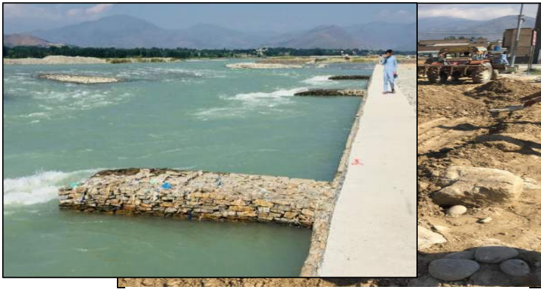
Fig. 64. Direct dumping of clayey material instead of boulders behind the wall. This issue needs to be addressed.
