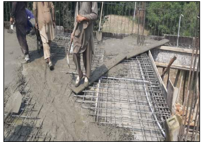
Fig. 12. Concrete pouring is in progress - GGPS Panam Dheri, Peshawar
