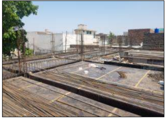
Fig. 20. Steel fixing in progress at Module M-4B - GHSS Nowshera Kalan
