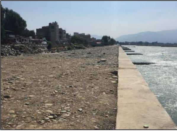
Fig. 61. View Fig.62. Three Stud were settling down due to flood in river needs safety measures to protect and rectify the executed work on river Swat
