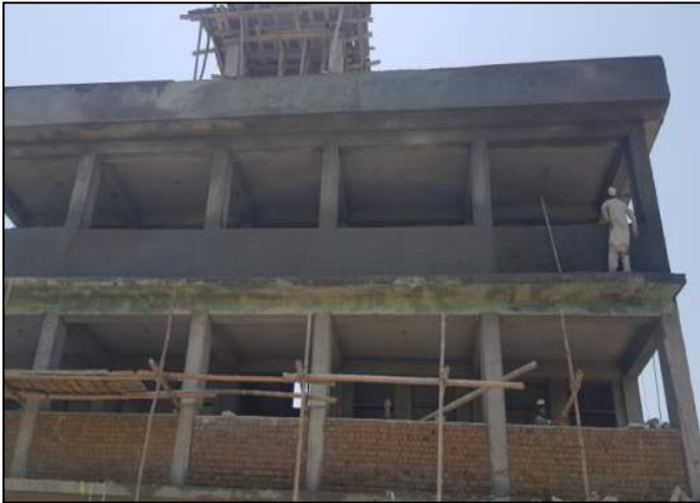
Fig. 15. Plaster in progress at parapet wall-GGPS Sadar Garhi, Charsada
