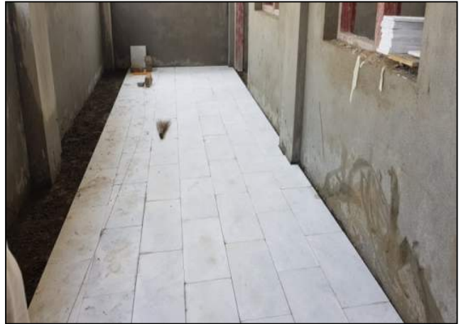
Fig. 16. Marble flooring in progress at 1st floor-GGPS Sadar Garhi, Charsada
