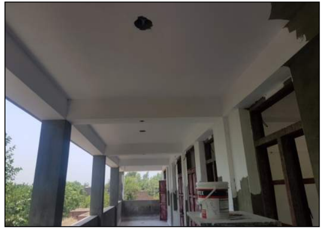
Fig. 14. Paint work in progress at first floor-GPS No.01 Katozai, Charsada
