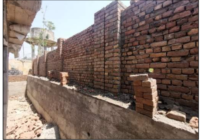
Fig. 42. Boundary wall works in progress at GGPS Naway Kalay, Swat
