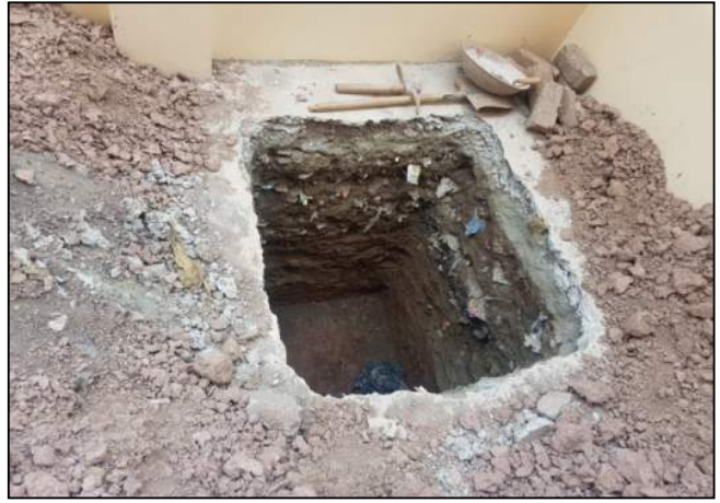
Fig. 26. Pit excavated for earthing -GGPS Aman Kot Nowshera
