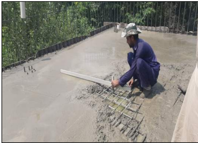
Fig. 11. Concrete during pouring is in progress - GGPS Panam Dheri, Peshawar
