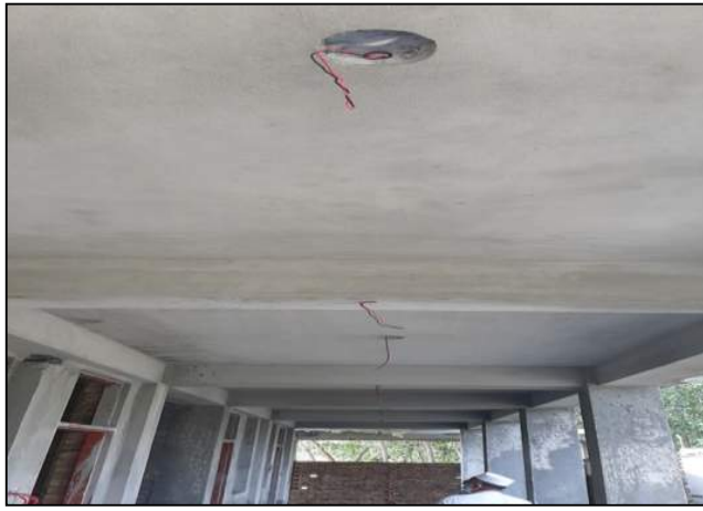
Fig. 07. Electric internal wiring is in progress – GPS Yari Koroona, Peshawar
