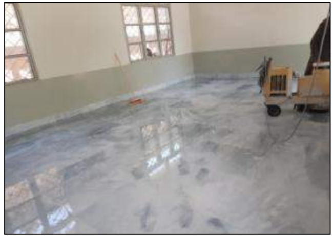
Fig. 22. Marble grinding in progress - GPS Toha, Nowshera
