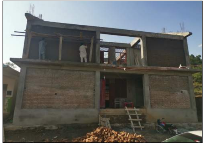
Fig. 44. External wall pointing works at T-7 of GGPS Daro Maira, Swat
