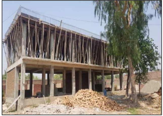
Fig. 32. View of Module M-6H-GHS Matani, Peshawar
