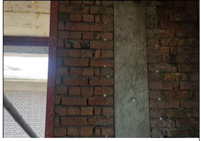
Fig. 02. Wire mesh fixed at column brick joints-GHS Pashtun Garhi, Nowshera
