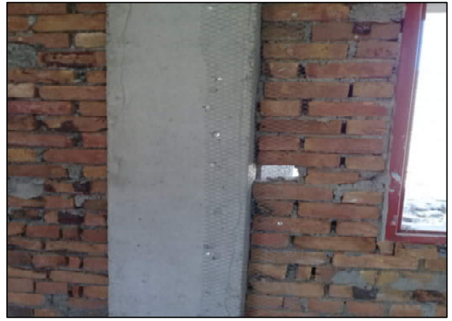
Fig. 08. Wire Mesh fixing in progress-GPS Yari Korona, Peshawar
