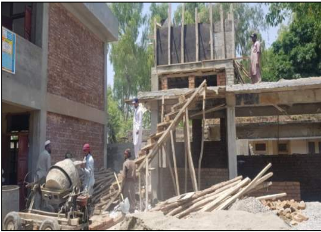
Fig. 13. Concreting in progress of OHWT-GPS no.01 Katozai, Charsada
