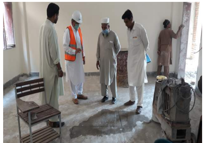
Fig. 06. COP-IQA inspecting terrazzo flooring at GHS Akbar Pura, Nowshera
