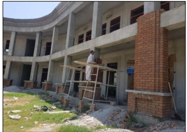
Fig. 04. Brick facing in progress at Block B - GHSS Akbar Pura, Nowshera
