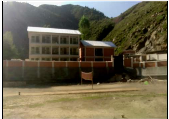
Fig. 58. Construction view of GHS Jan Bhatti, Dir Upper
