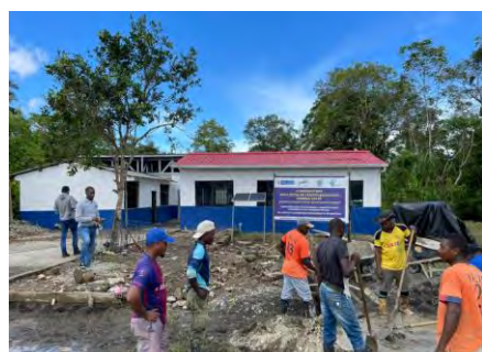
Community of the village of Yalté participating in the construction process.
