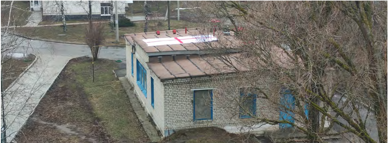
A technical building at the Iziium Central City Hospital, which was damaged in at least three attacks in March 2022, showing the red cross placed on its roof to indicate its status as a medical facility. Photo captured by hospital director Dr. Bohdan Berezhnyi in Feb/Mar 2022.
