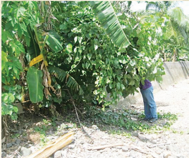
Rehabilitation of Existing Flood Control Project (Pandan, Catanduanes)
