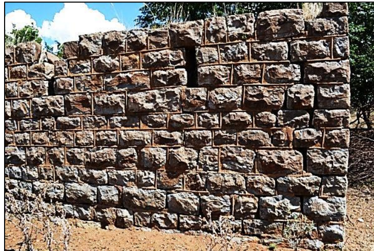
Figure 5. Detail of stone masonry work on the dolomite outbuilding (Photograph: M. Naude 2013)
