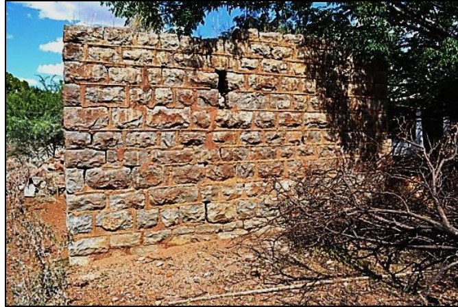
Figure 4. Gable end of the dolomite structure without roof (Photograph: M. Naude 2013)
