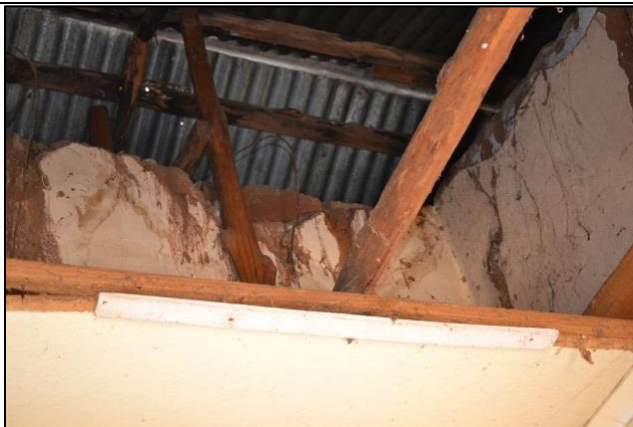
Figure 40. The interior walls were also elevated and the roof structure was replaced over time (Photograph: M. Naude 2013)
