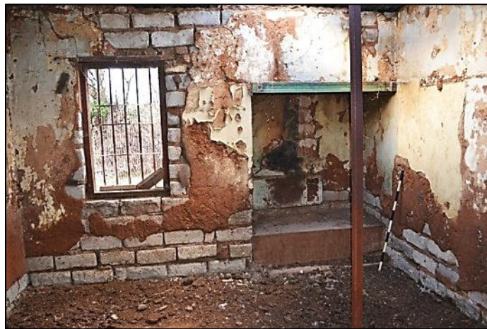
Figure 12. Hearth in the kitchen of the workers dwelling (photograph: M. Naude 2013)
