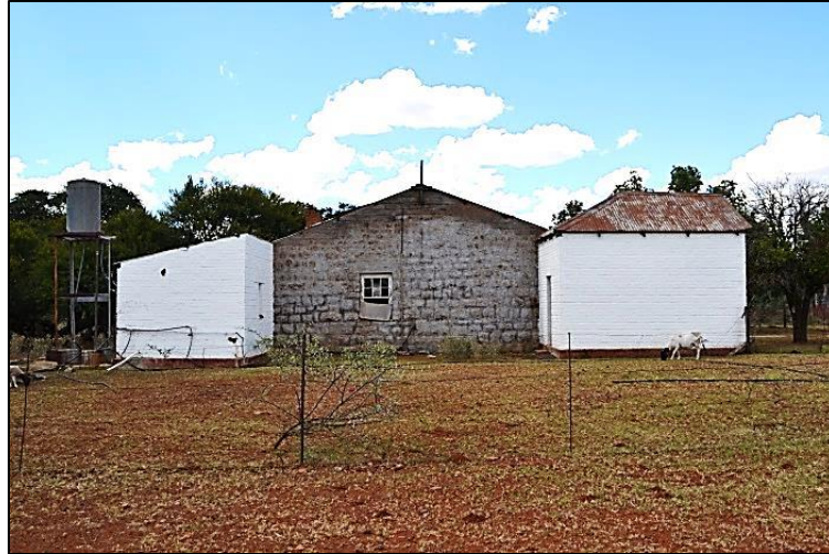
Figure 23. Side elevation with exposed dolomite gable end and two stoepkamer additions (Photograph: M. Naude 2013)
