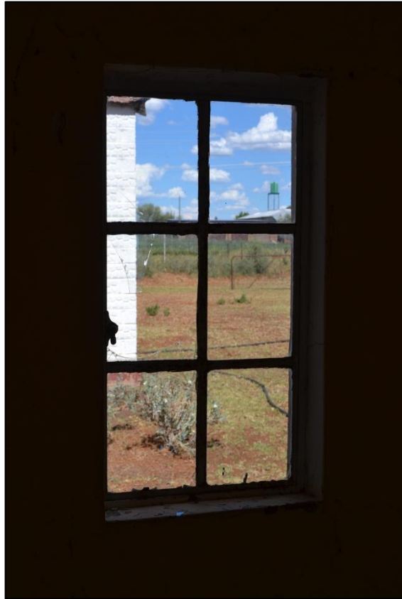
Figure 31. Steel frame window (Photograph: M. Naude 2013)
