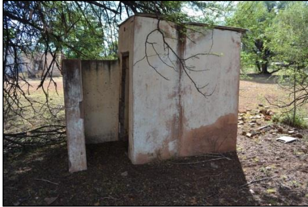
Figure 6. Side elevation of the detached outdoor privy (Photograph: M. Naude 2013)
