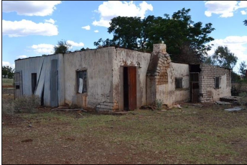
Figure 5. Separate workers dwelling in the backyard
