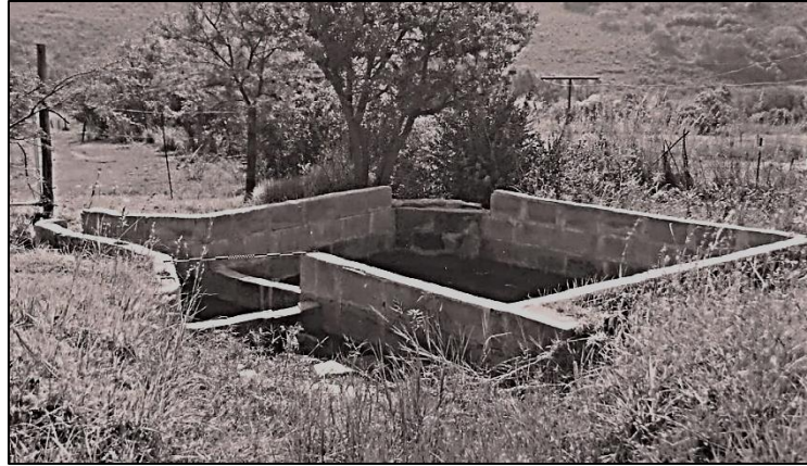
Figure 9. More formal water furrow distributor dam constructed with cement blocks (Photograph: M. Naude 1988)
