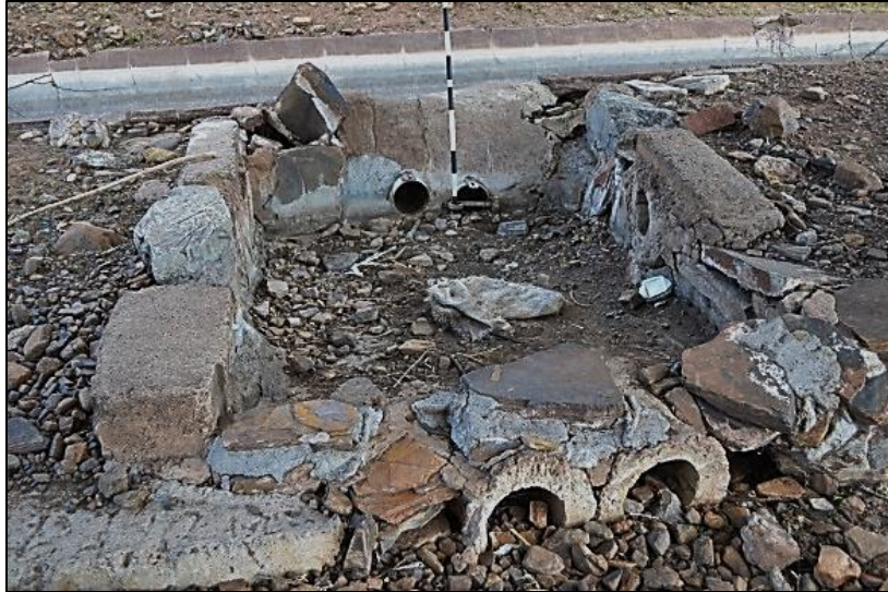
Figure 7. Furrow distributor dam adjacent to the dam from where water was irrigated into the gardens and orchard (photograph: M. Naude 2013)
