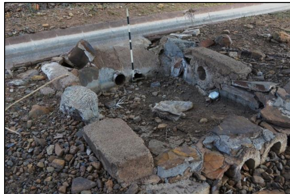
Figure 14. Water furrow distributor dam with furrow at the back and various outlet pipes in front (Photograph: M. Naude 2013)
