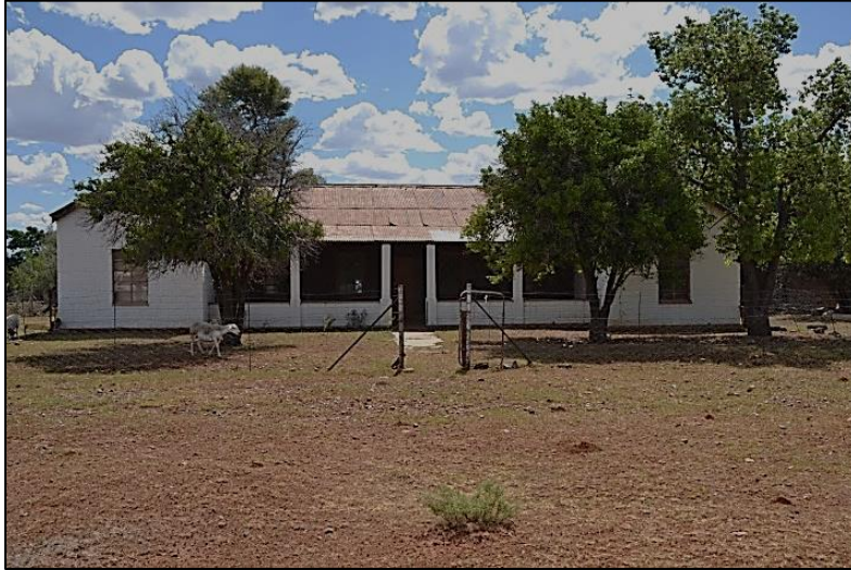
Figure 11. Front elevation of the principal dwelling - view from the street
