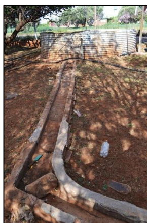
Figure 16. Open water furrow leading directly from the corrugated iron water reservoir (photograph: M. Naude 2013)
