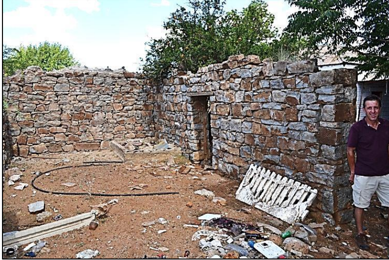
Figure 3. Interior of dolomite stone outbuilding
