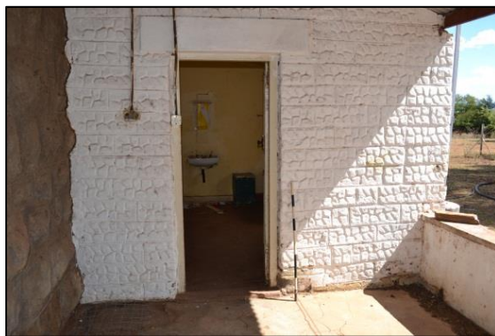
Figure 42. One of the stoepkamers on the back verandah that was later added that differs from the original core dwelling constructed with stone masonry (left) (Photograph: M. Naude 2013)
