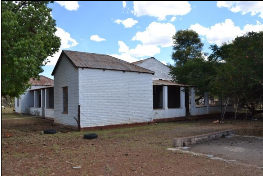
Figure 1. Side elevation of the dwelling with stoepkammer in the centre and verandahs on both sides
