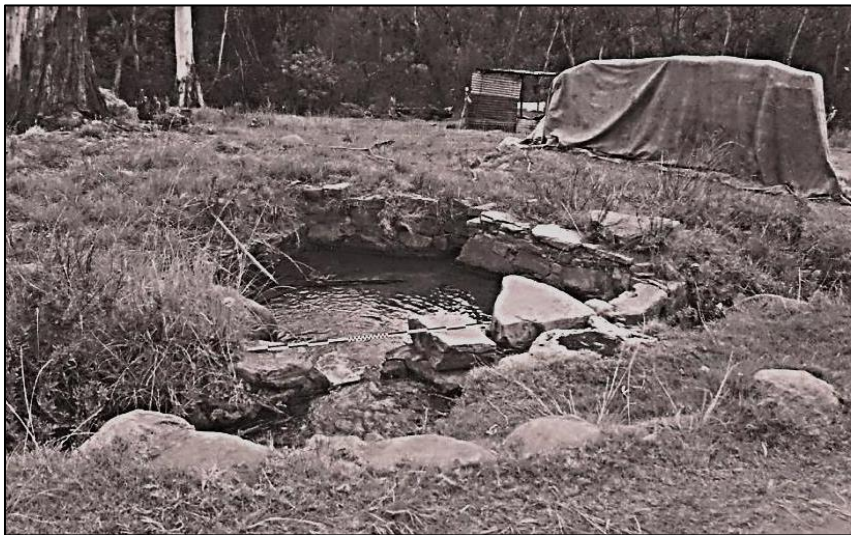
Figure 8. Simple water furrow distributor dam constructed with stone walling
