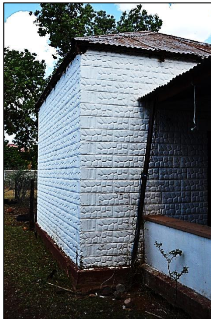
Figure 18. Prefabricated cement bricks mimicking the texture of stone, used for all the later additions and stoepkamers (Photograph: M. Naude 2013)
