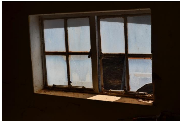
Figure 30. Interior of steel frame window in bath room (photograph: M. Naude 2013)
