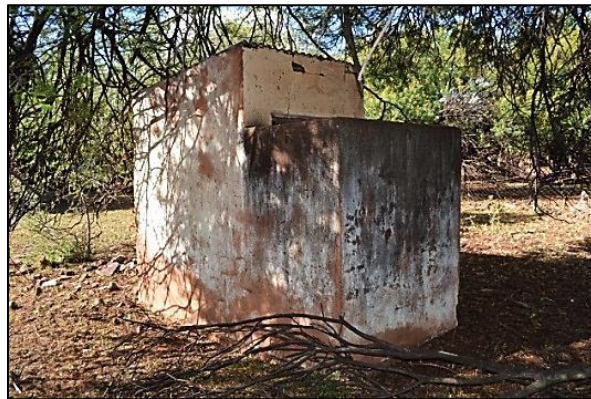
Figure 7. Protecting wall of semi-open outdoor privy (photograph: M. Naude 2013)
