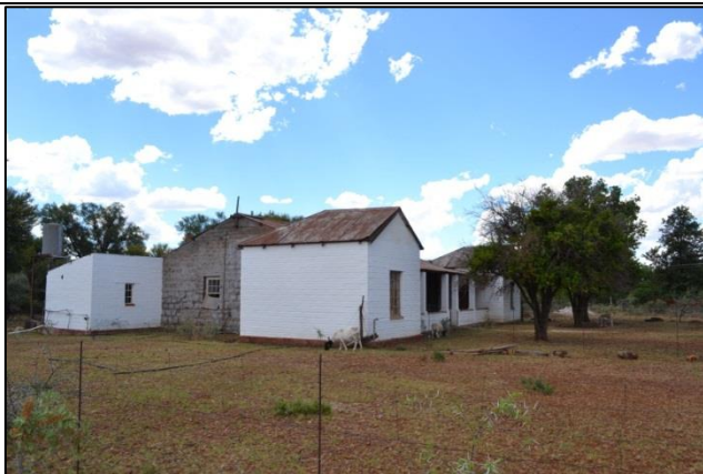
Figure 41. The later additions and extensions are clearly defined by the whitewashed rooms and supporting columns of the front verandah (Photograph: M. Naude 2013)
