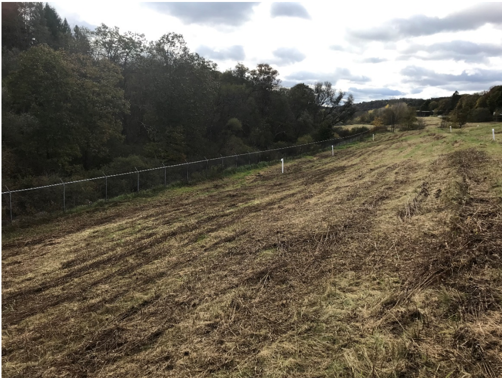
Gas vents and fence along the South Branch of Bear Creek
