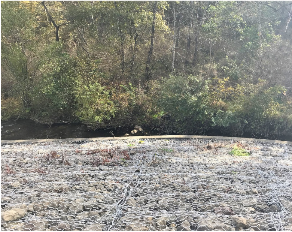
Dike along Eastern site boundary
