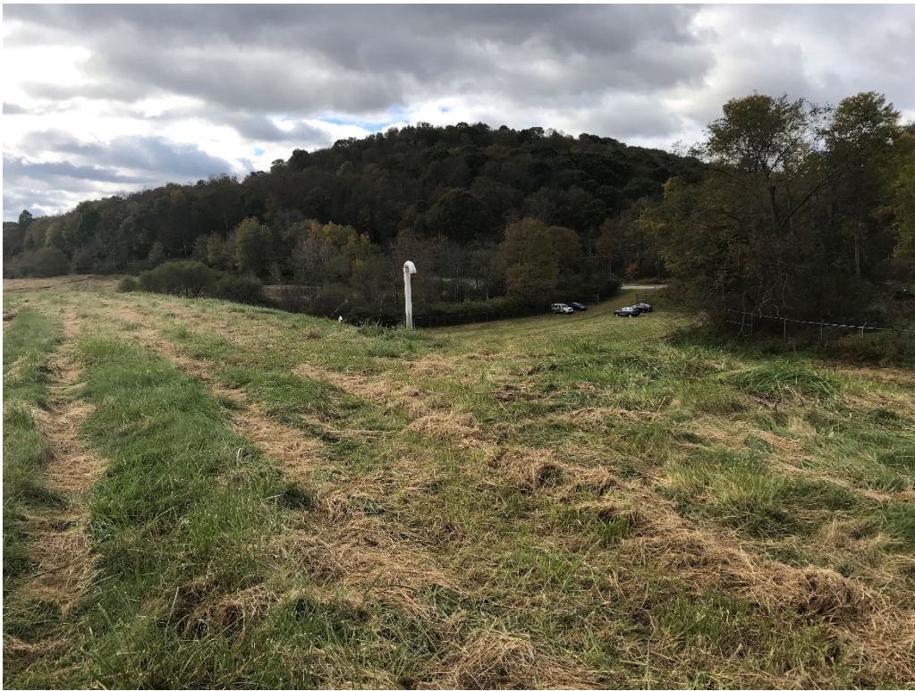
Gas vent, looking toward site entrance
