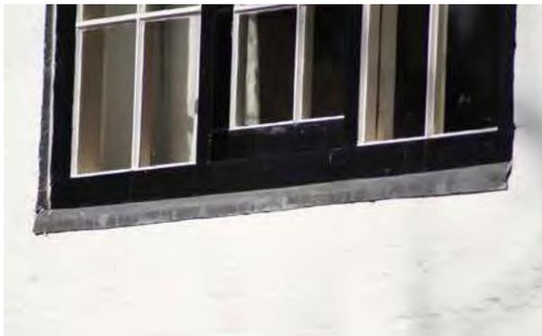
A piece of lead has sometimes been added to protect the brickwork beneath (left and bottom left - 63 Main Street and stables at The Hall).
