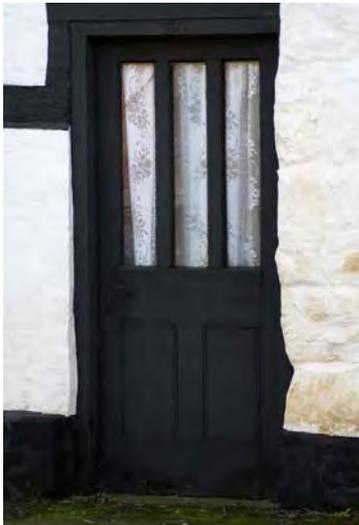
Left - panelled door with pair of flush bottom panels incorporating bead mouldings and three glazed panels separated by muntins (54 Main St).
