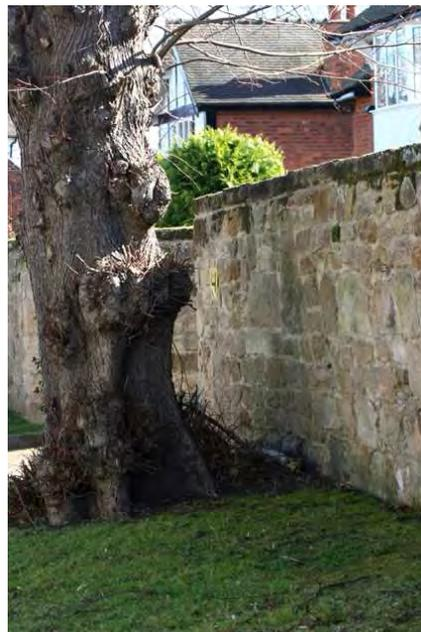
Left and far left - tall, mortared rubble gritstone walls fronting Main Street incorporate either triangular, chamfered or flat copings.
