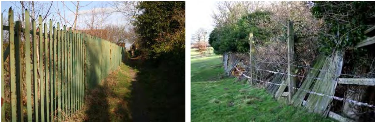
The northern fenced boundary to Kings Newton Hall grounds has partially collapsed and is in poor condition (pictured above right). It incorporates concrete stanchions, timber posts and rails and timber cladding, all repaired in barbed wire. The unkempt appearance detracts from the rest of the park and garden.
