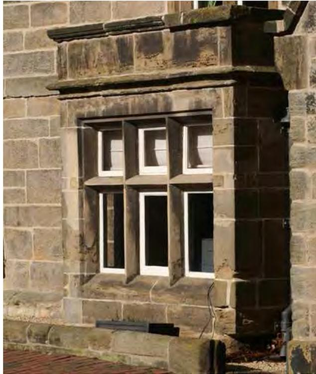
Above - bay window at Chantry House, a 19th century addition, incorporating chamfered mullions and transom, plain casements and parapet with moulded cornice.
