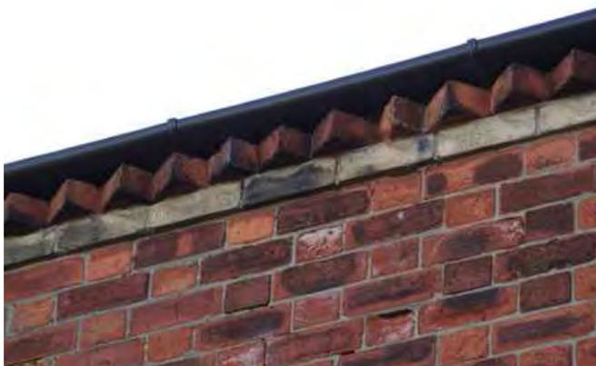
There are several types of decorative brick eaves within the village. Some incorporate brick corbelled out in a “dentilled” or “sawtooth” pattern
