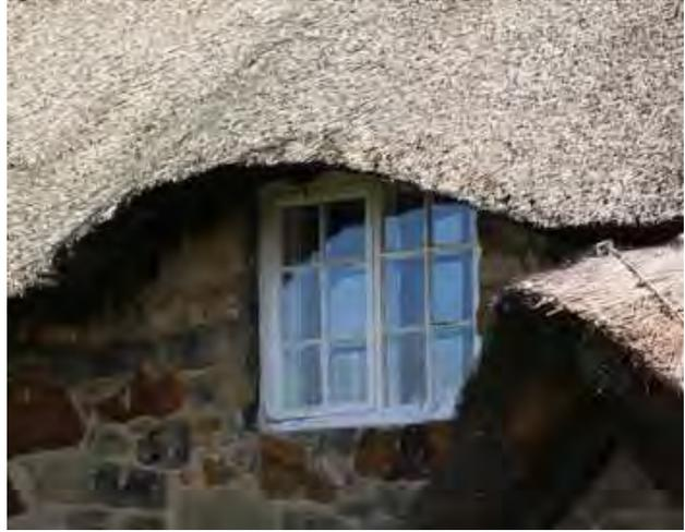
Left - along Main Street there are many examples where small gables with overhanging eaves and fascia boards were added, when the buildings were re-roofed around the turn of the 20th century. The tiled roofs replaced thatch. The only example of a thatched roof is at Manor Oak Cottage (above). The eyebrow dormer within the thatch has much softer lines than the tiled gables.
