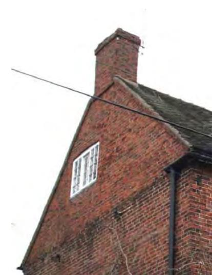
Left - A typical gable end chimney (Elms Farm, Trent Lane, 1801-3) with plain oversailing courses at the top. Note how the projecting string course under the tiles on the roof verges is carried across the base of the chimneystack.
