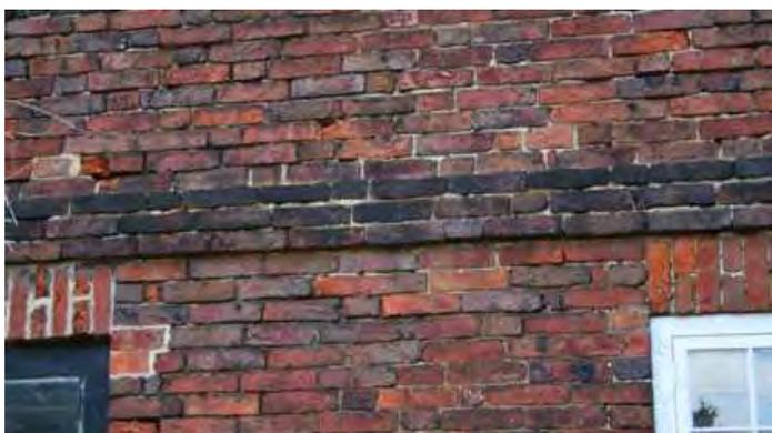
Above centre - raised brick band with “dentilled” bricks, and stone quoins, at 32 Trent Lane. Above - 18th century raised horizontal brick band (the stableblock to The Hall).
