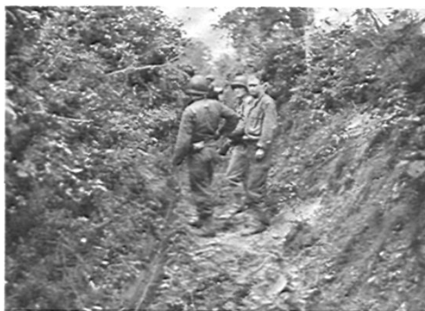
Laying wire among the hedgerows near St. Lo.
