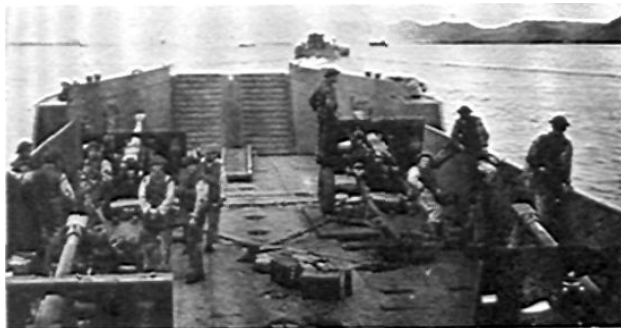
Highly effective fire is delivered during the landing by field artillery firing from LCTs. Britain's 25-pounder, with muzzle brake, is one of the weapons found highly suitable for such use.
