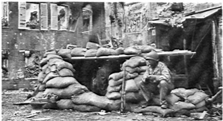
Outposts should have protection and concealment. This AT gun is well equipped with both, even to overhead cover to keep falling bricks off the crew.
