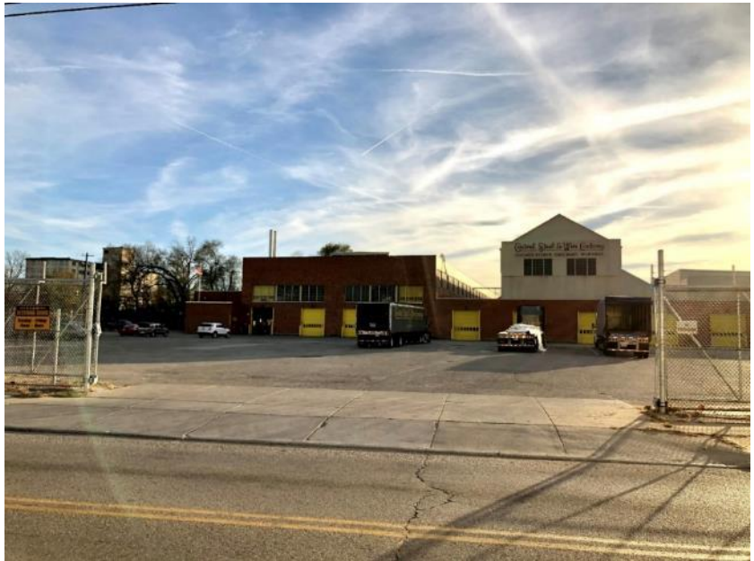
CENTRAL STEEL AND WIRE, LOOKING SOUTHWEST FROM TOWNSHIP AVENUE
