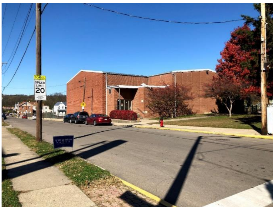
ELMWOOD PLACE ELEMENTARY SCHOOL BUILDING, FROM VINE AND MAPLE STREET INTERSECTION
