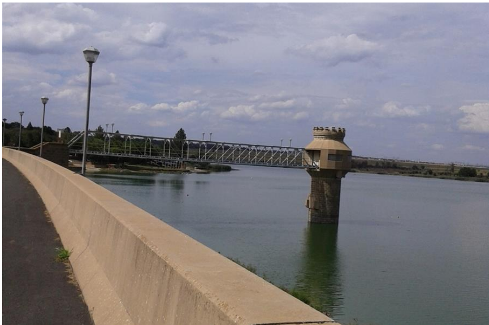
Figure 4.8: The ground wall of the Rietvlei Dam Photo: Author (9 December 2015)
