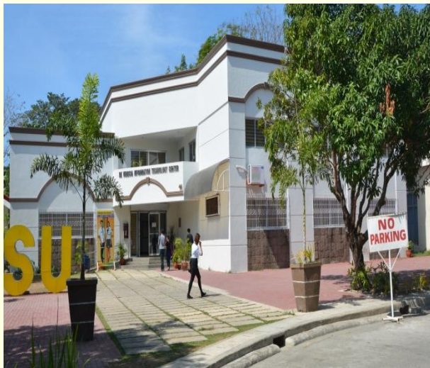
Repair of Convention Hall – Php3.5M Lingayen Campus
