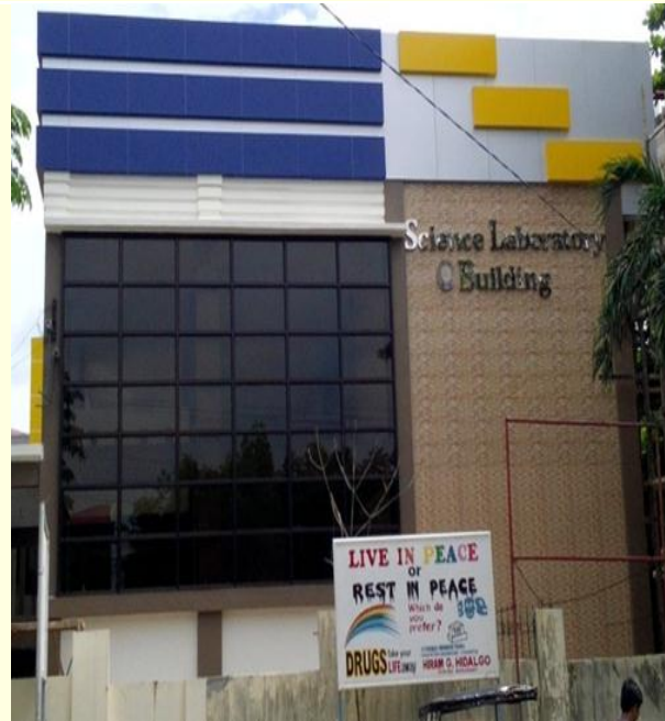
New Science Laboratory Building - Php23.308M Lingayen Campus
