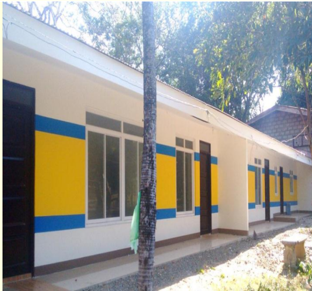
Repair of Dormitory – Php2.4M Bayambang Campus
