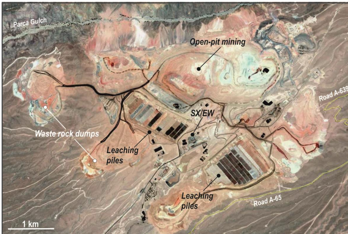
The Cerro Colorado mining-metallurgical complex. SX/EW: "Solvent Extraction-Electrowinning".
