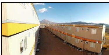
Collahuasi: Camp Pioneer expansion consisting of 3 Modular Buildings of 2 and 3 stories with metal staircases on the outside (ATCO Sabinco 2017).
