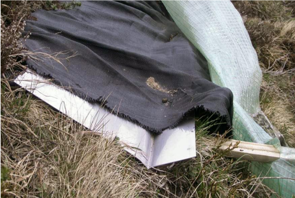
Fig. 30 > Flattened sediment trap due to snow movement after the winter of 2007/2008
