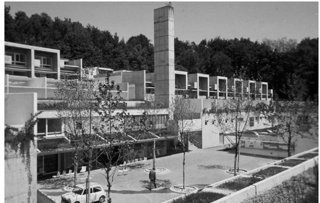
03 Central square immediately after completion. The horizontal streets and pathways and the perpendicular stairs lead up to it; they all lead to the square tangentially, not axially. The shop, the club-room and the laundries are directly connected to the square. On their way to the public transport stations or to the parking garage most of the inhabitants cross the square. © Archive Atelier 5 . Photo by Albert Winkler, 1960s.
