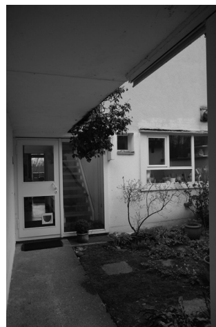
05 Courtyard of the broad type of houses. It is private, but orientated to the pathway, the public space. Beyond the outside door (many inhabitants normally leave it open) the view opens onto the courtyard and to the northern façade. A covered path leads to the entrance. Note the differentiated manners of mounting the windows (from outside, flush mounted, from inside). © Bernhard Furrer, 2012.
