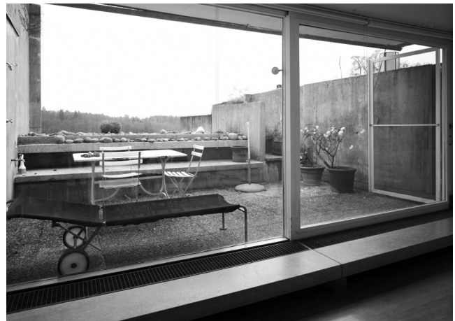
10 Solarium of the broader type of houses. The room behind the solarium opens wide to the outside with a concrete step that hides the convection heater and sliding windows with very slim frames. Towards the south a trough with plants forms a limit to the solarium, a sort of recess permits an overview of the Estate and the landscape. In accordance with the guidelines, covering of the solarium is not allowed anymore. © Archive Atelier 5 . Photo by Nikolaus Schletterer, 1960s.
