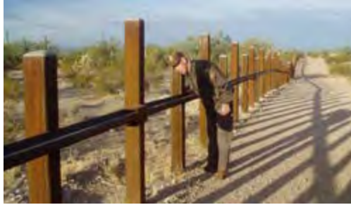
Photo 1: Vehicle barrier in Organ Pipe NM. Photo credit: National Park Service
