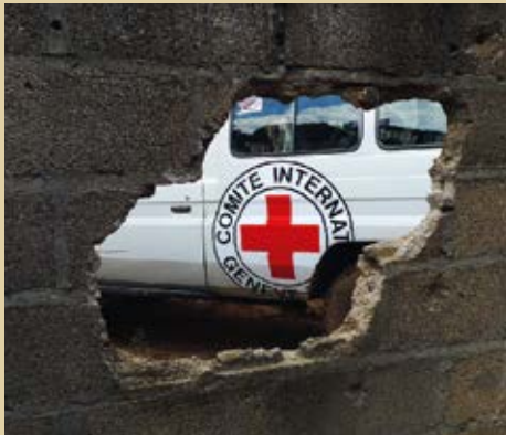
A house destroyed by an armed group, in the background an ICRC land cruiser. Tolima department, municipality of Ovejas-Sucre, district of Pijiguay, Colombia, 2022.
