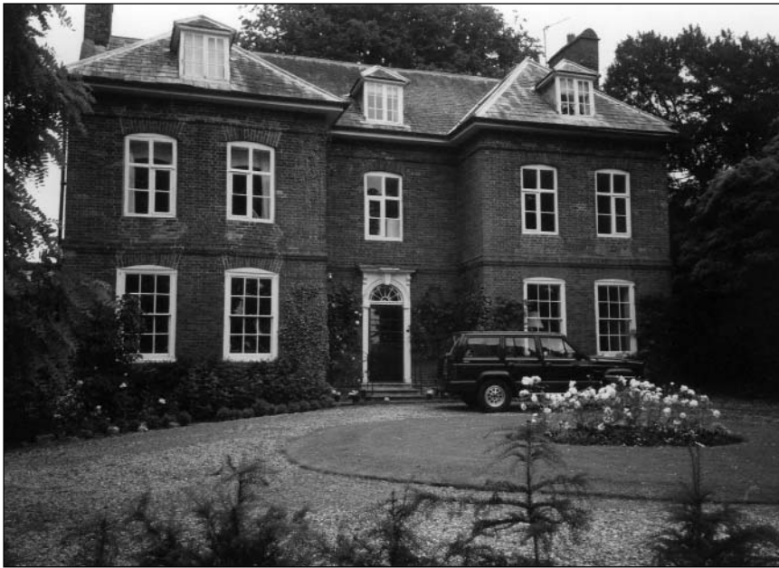
The former rectory, build by the Rev Chapman Dolby early in the 18th century
