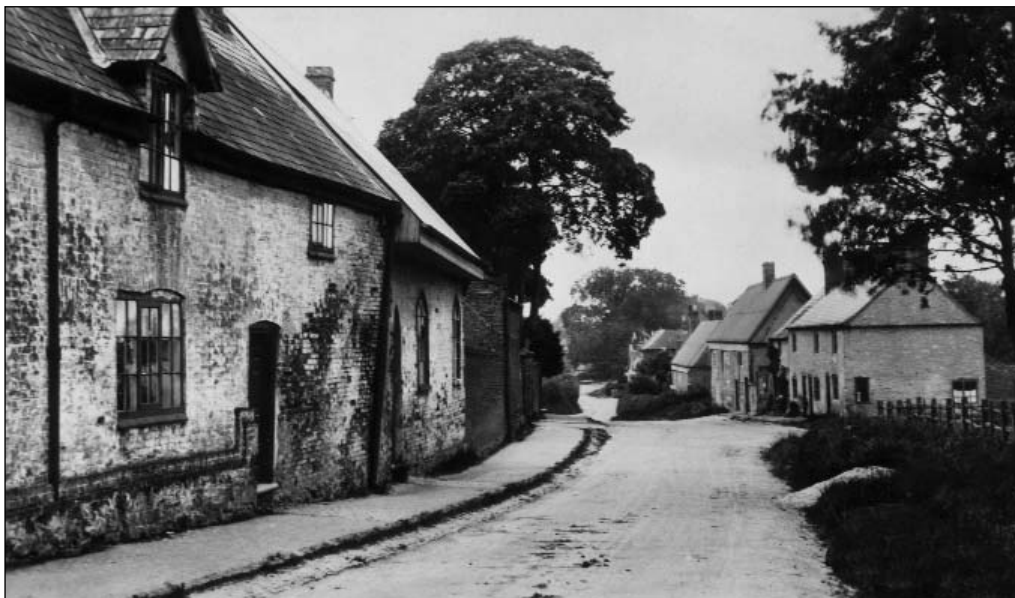
The old meeting room, at the far end of the building, with two arched windows. It was demolished in 1973
