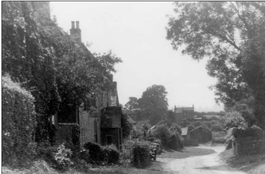
View down Back Lane
