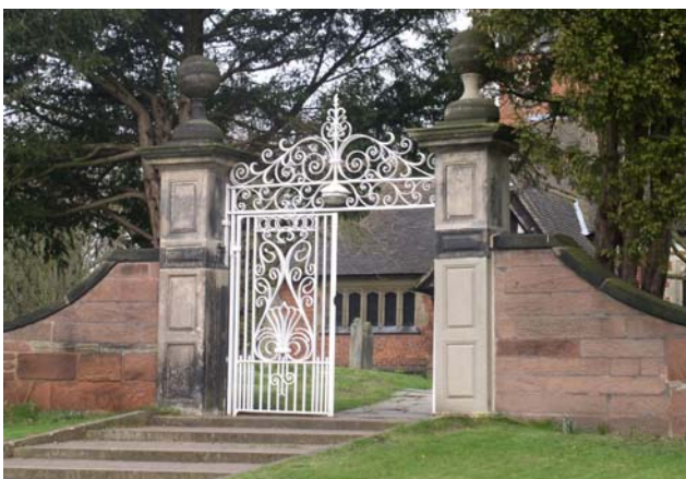
St Mary Church gate and gate piers
