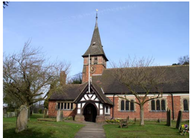
St. Mary's Church, South elevation
