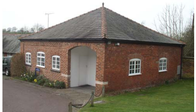
The Mews – former stabling
