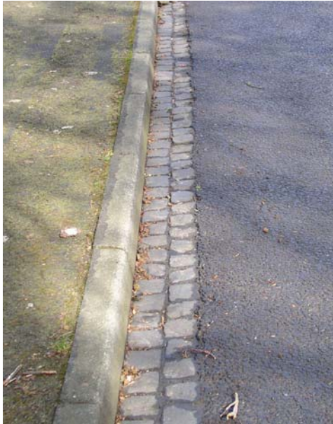
Setts along highway edge adjacent to the Church
