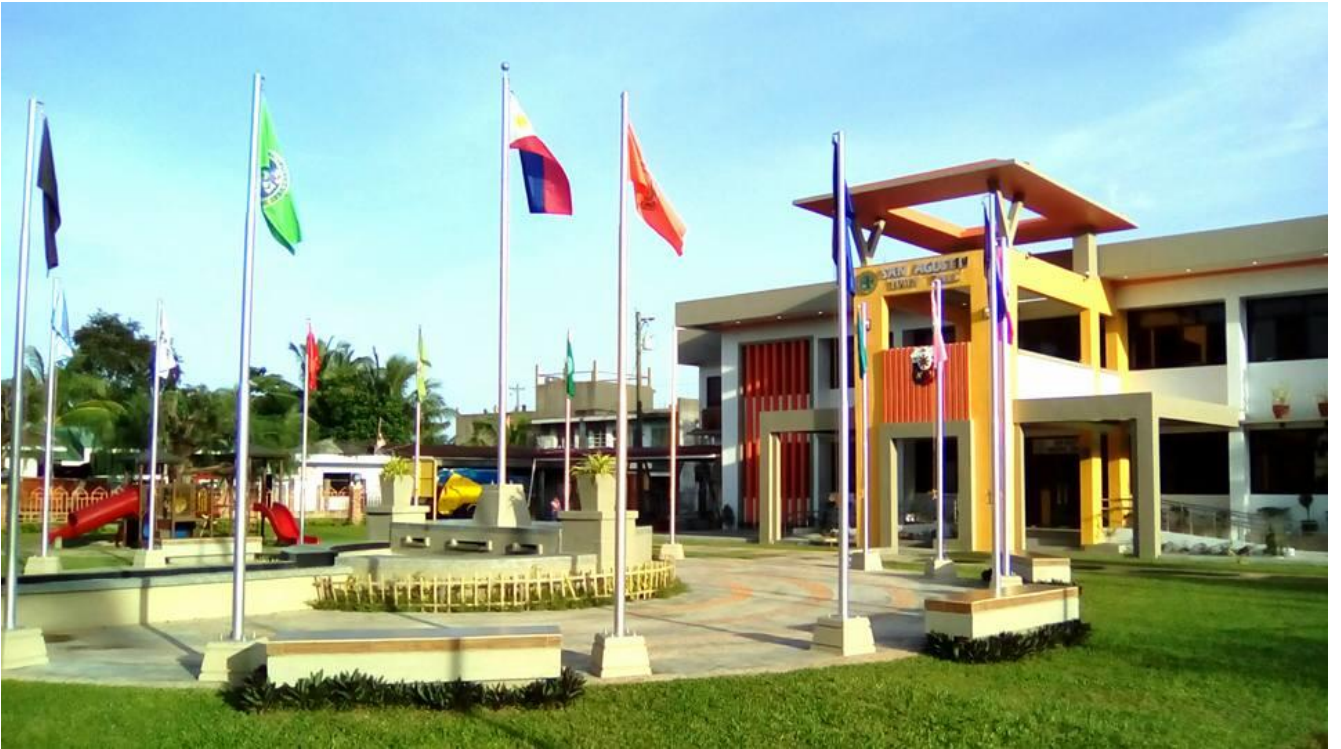
Figure: San Agustin, Municipal Hall Facade
