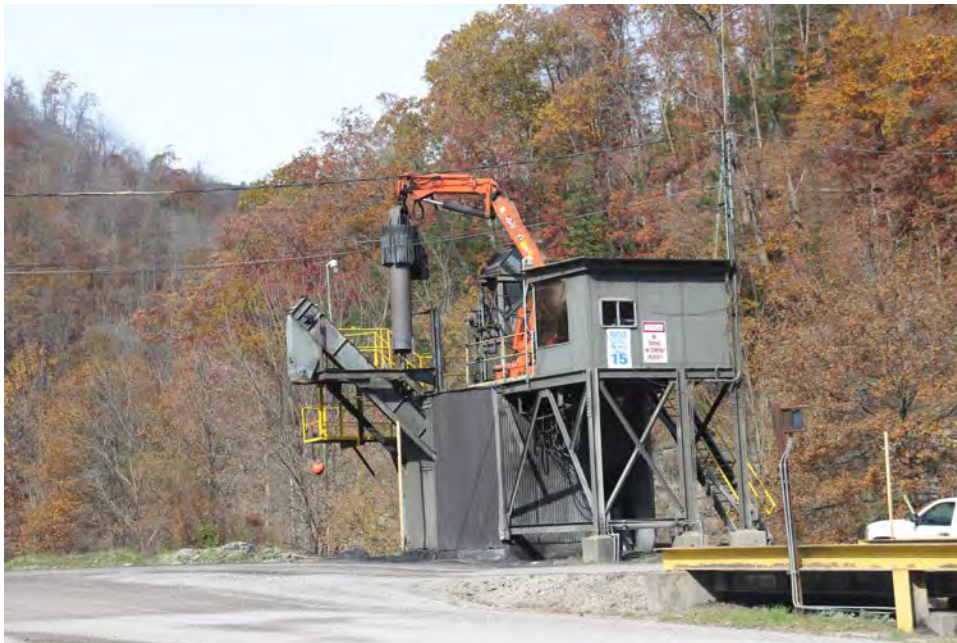
The truck scale with its coal sampler. The suction pipe is lowered down into the truck's load of coal to draw a sample to verify that it is the correct quality of coal. The conveyor belt delivers the sampled coal into a truck for removal to the coal stockpile area.
