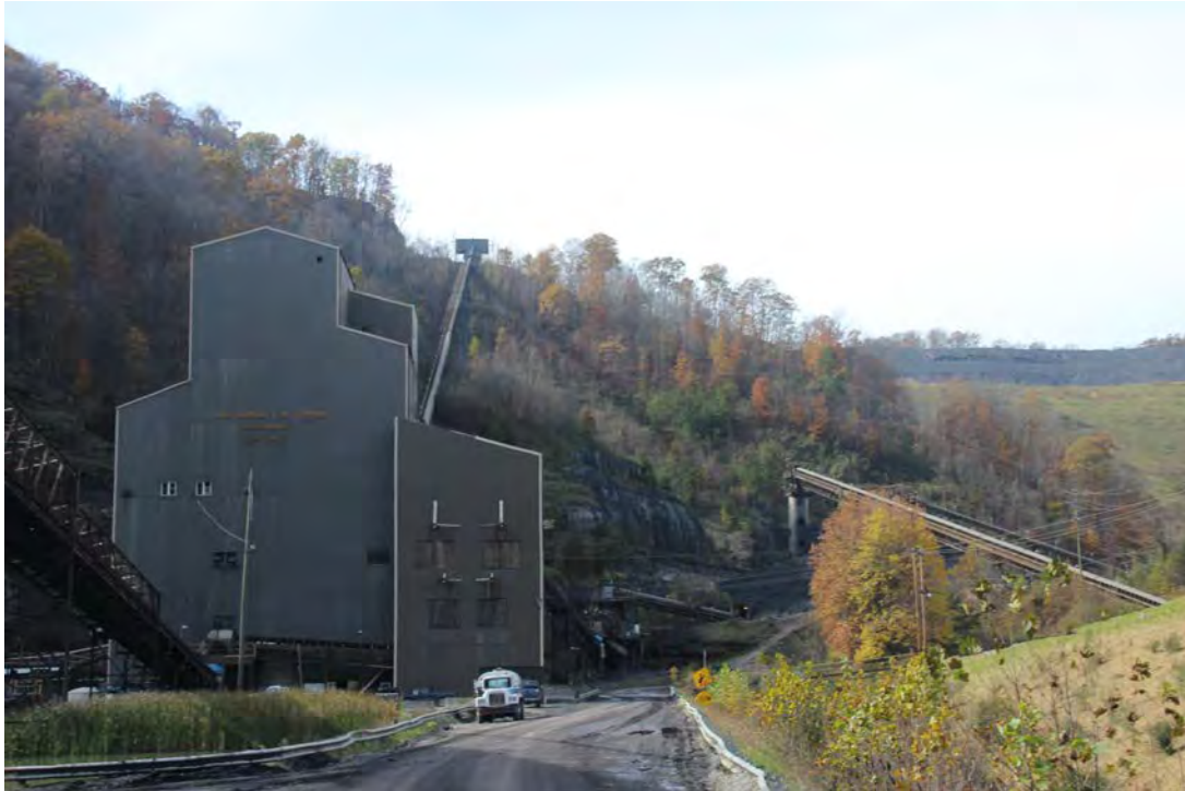
Above and below are views of the wash plant looking at its north side. The conveyer belts are carrying washed coal from the plant to the storage area.
