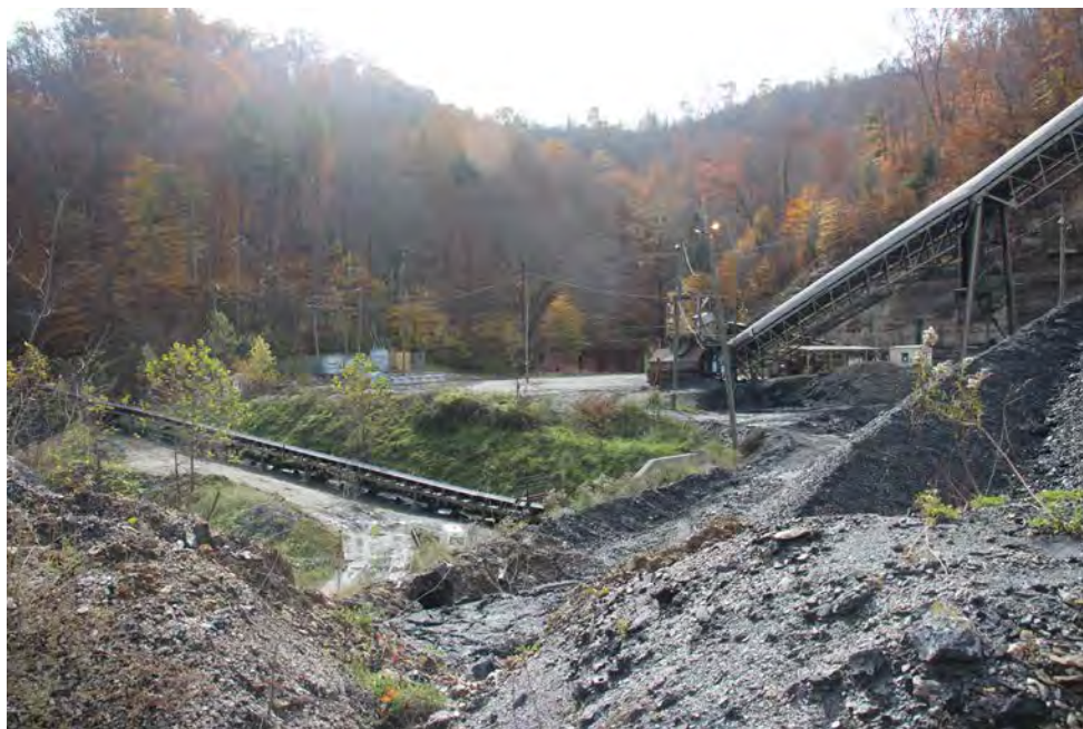
Conveyor belts snake through the property carrying coal to the wash plant from various coal veins that are being worked on the property.
