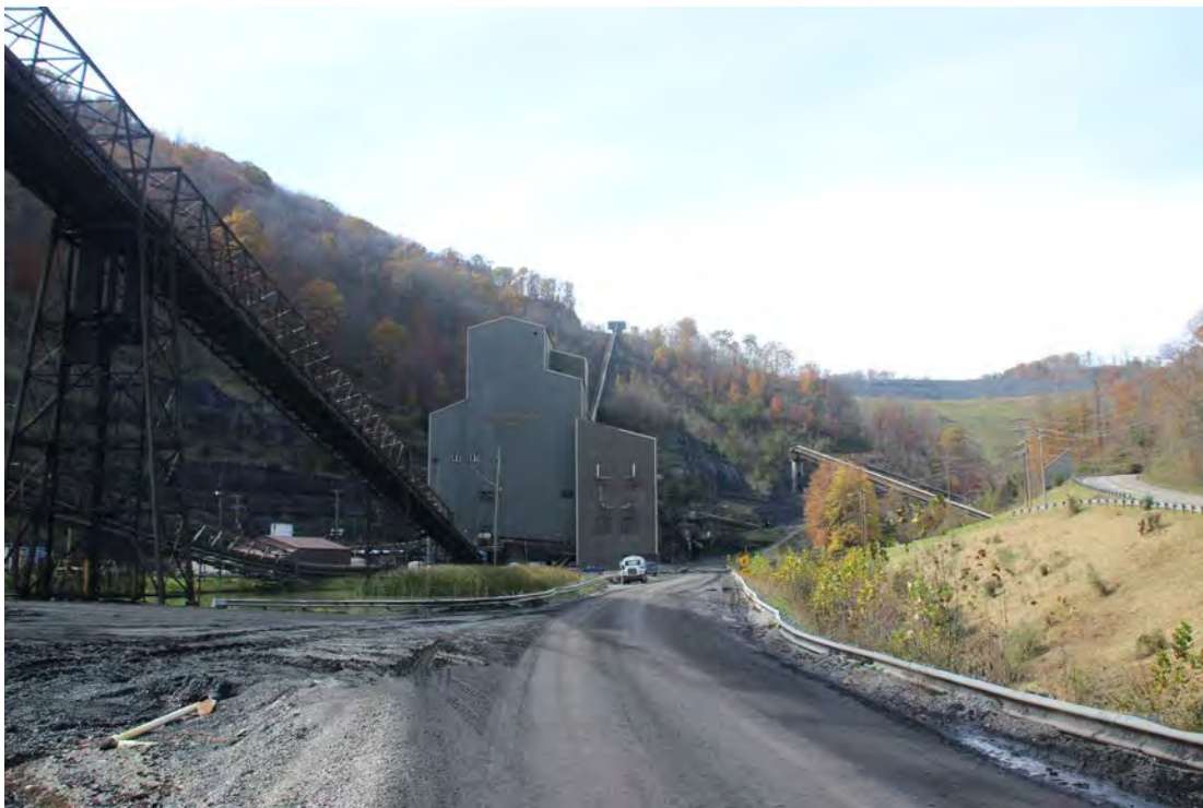
Above and below are views of the wash plant looking at its north side. The conveyer belts are carrying washed coal from the plant to the storage area.
