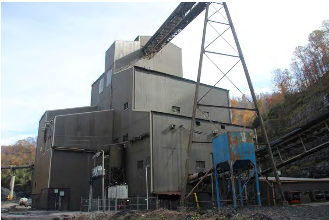
A close-up of the wash plant. Here the coal is floated in water to remove impurities, for the power plant contract calls for coal of a certain BTU with less than .05 percent non-burnable material mixed in with the coal.
