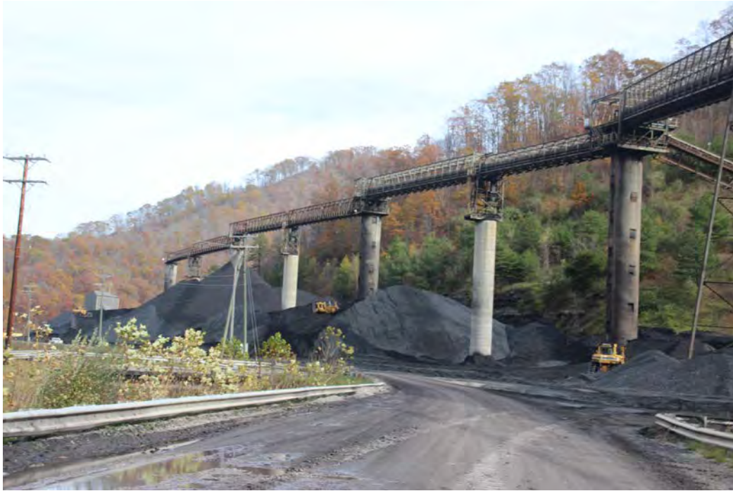
Above and below is the coal storage area. Underground augers carry the coal from here to a conveyor belt that leads to the train flood loading tippie. Note in the photo below the D9 bulldozer working the coal pile. Coal is dumped into the top of the cylinders and falls out to the storage area through window cut in the cylinder walls.
