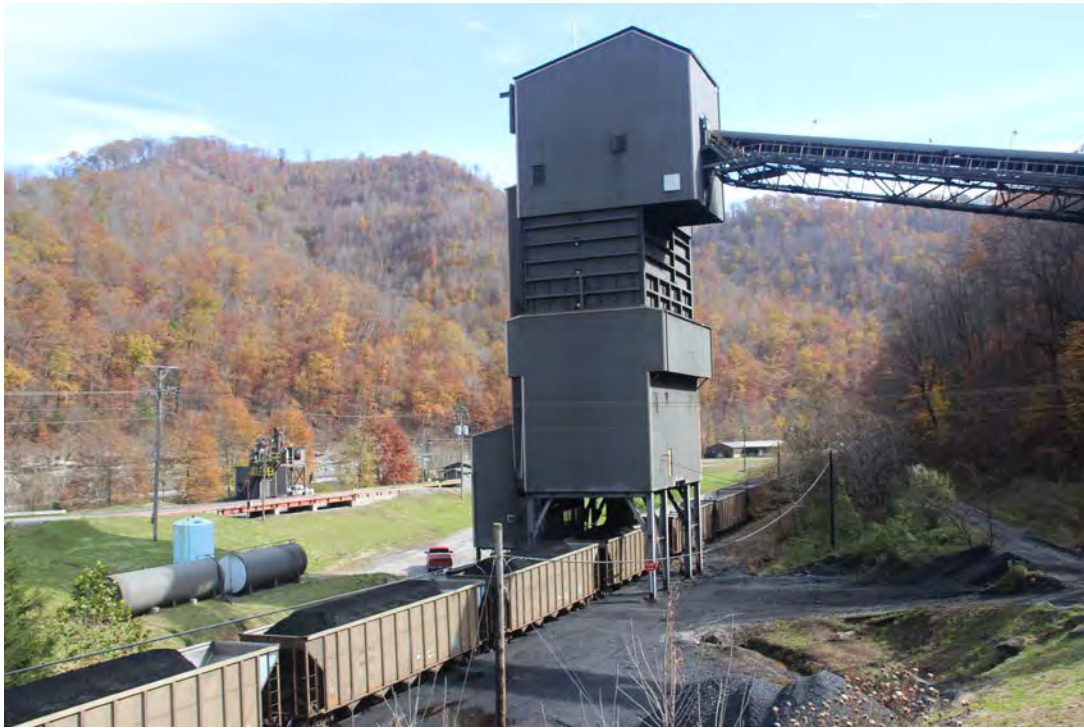
A view of the flood loader. A balloon track leads to the flood loader from the CSXT track. One leg of the balloon track can be seen up against the cliff wall beyond the telephone pole.
