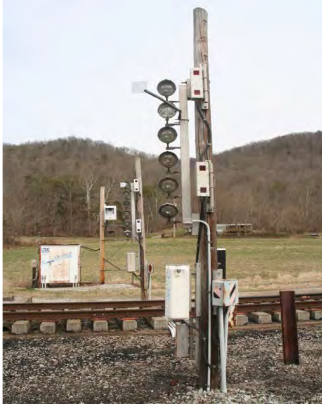
Lights for lighting up the car's reporting marks as it rolls over the scale and the video cameras that transmit the image to the Jacksonville Operation Center
