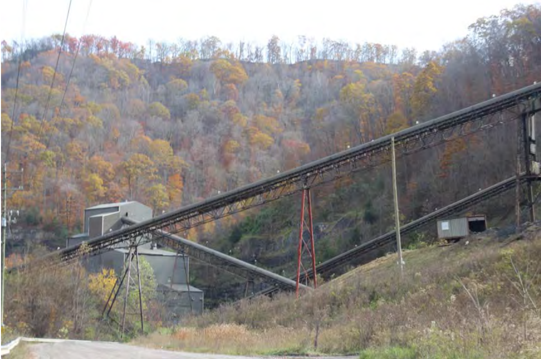
The conveyor belt is nearing the end of its journey, for the wash plant is visible in the lower left. The view is toward the southside of the wash plant.
