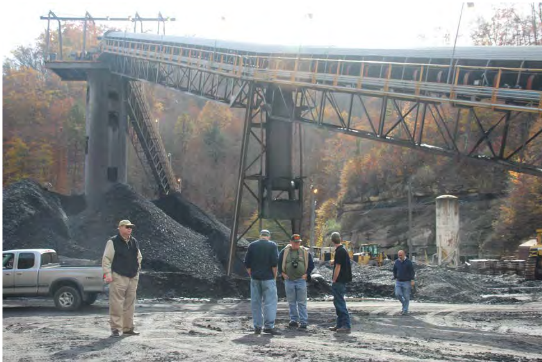
The above conveyor belt carries the newly mined coal to this stockpile area. From here the coal is sent to the wash plant. The ground is black mud.
