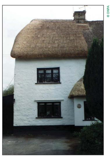
Fig 7 Thatched roof with ridge laid flush in traditional manner
