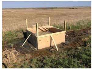
**Photo #11** View (looking southeast) of installed wooden piling walls around cased borehole (May 2016).
