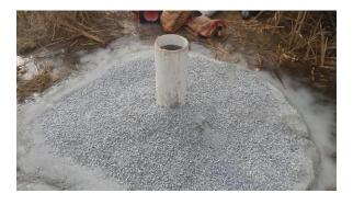
**Photo #6** View (looking west) of borehole after being grouted and cased (March 2016).
