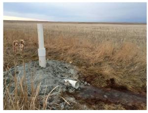
**Photo #9** View (looking northeast) of second casing and piping inserted for water flow to help with erosion (March 2016).
