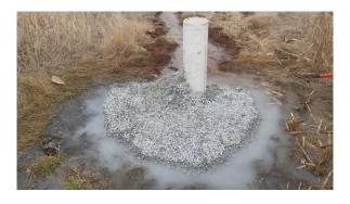
**Photo #5** View (looking south) of borehole after being grouted and cased (March 2016).
