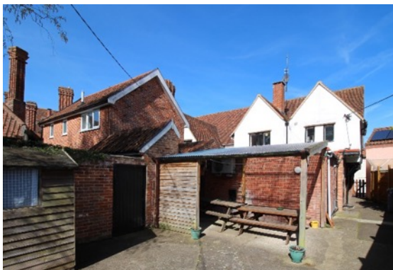
South elevation of the Social Club
