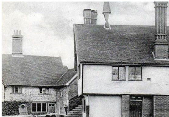
Detail of a c1900 postcard of the Guildhall and Club, at first sight unchanged, but Shaw's bellcote and steps have now gone, and the windows of the Georgian cottage behind have been radically altered
