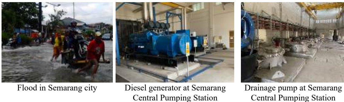
Figure 2-28 Flood in Semarang City, Drainage Pump, Power Generation System
