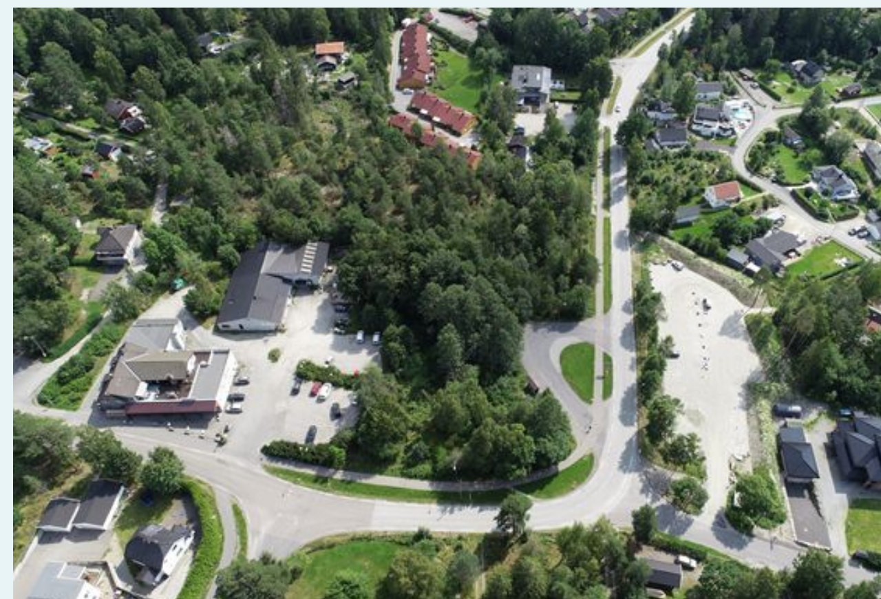
Skogheimkrysset / The Skogheim Junction. Drøbakveien disappears at the top of the image.
